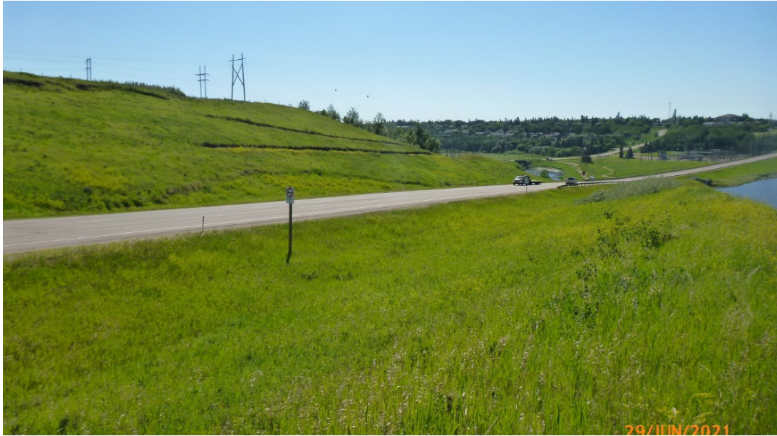
Photo 2 Ditch bottom and toe roll of the slope east of Hwy 41:02. Recent movement difficult to determine due to height of the vegetation on the slope. Photos taken June 29, 2021 looking northwest.
