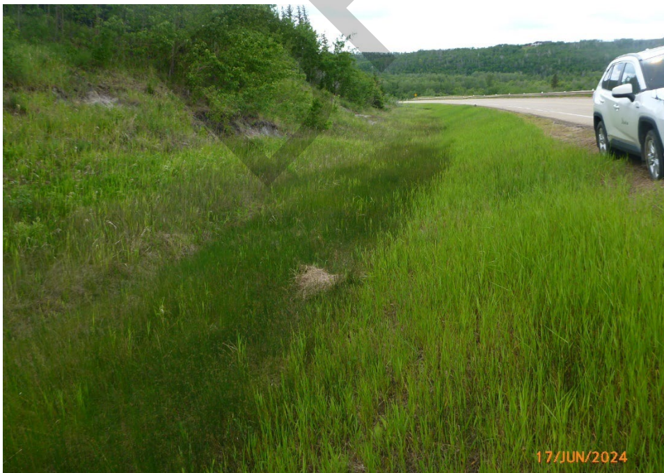
Photo 6 Area of dense vegetation in south (eastbound) lane could indicate an area with poor drainage and surface water infiltration into the highway embankment (overall, the ditch is graded to facilitate positive drainage). Photo taken June 17, 2024, facing west.
