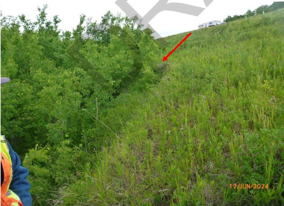
Photo 4 Minor scarp (indicated by red arrow) located approximately 10 m downslope (north) of the guardrail. The minor scarp is approximately 1 m in height. Photo taken June 17, 2024, facing southeast.
