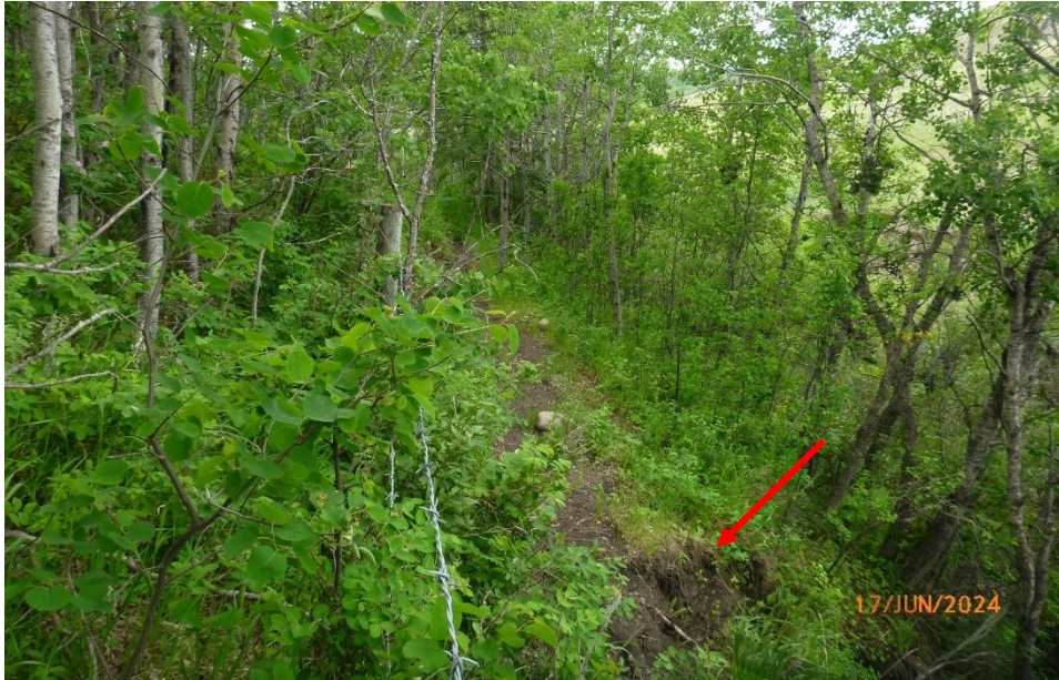
Photo 6 Area of dense vegetation in south (eastbound) lane could indicate an area with poor drainage and surface water infiltration into the highway embankment (overall, the ditch is graded to facilitate positive drainage). Photo taken June 17, 2024, facing west.
