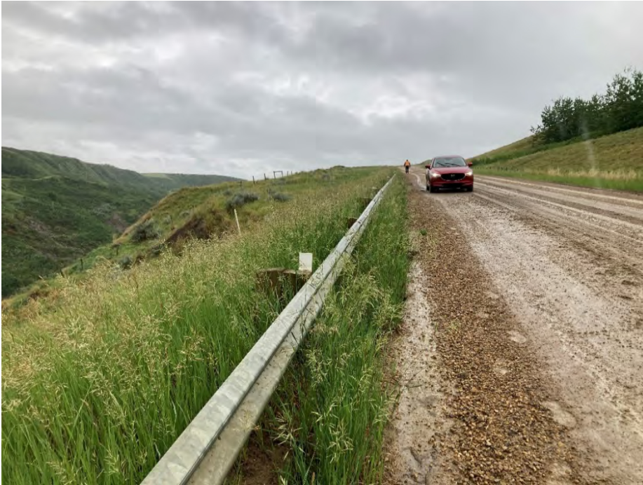
Photo 2 Small amount of erosion adjacent to the guardrail south of Hwy 569. Photo taken June 24, 2021 facing east.
