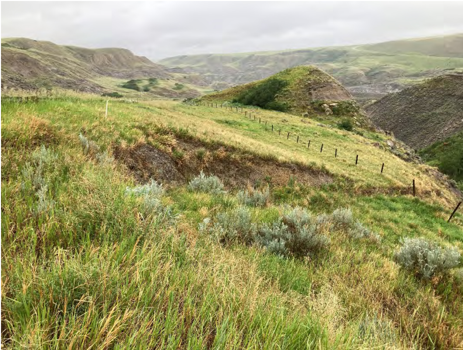
Photo 4 Backscarp of the slide south of Hwy 569. The slide does not appear to have progressed since the inspection in 2020 and appears to be inactive, excluding some minor erosion on the near-vertical backscarp. Photo taken June 24, 2021 facing north.
