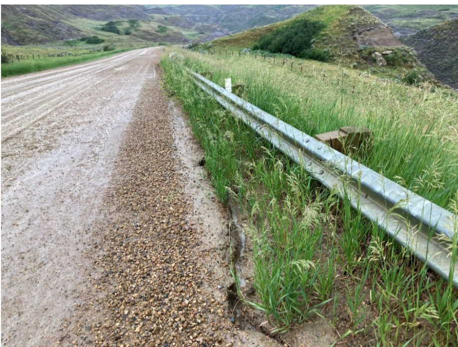
Photo 2 Small amount of erosion adjacent to the guardrail south of Hwy 569. Photo taken June 24, 2021 facing east.
