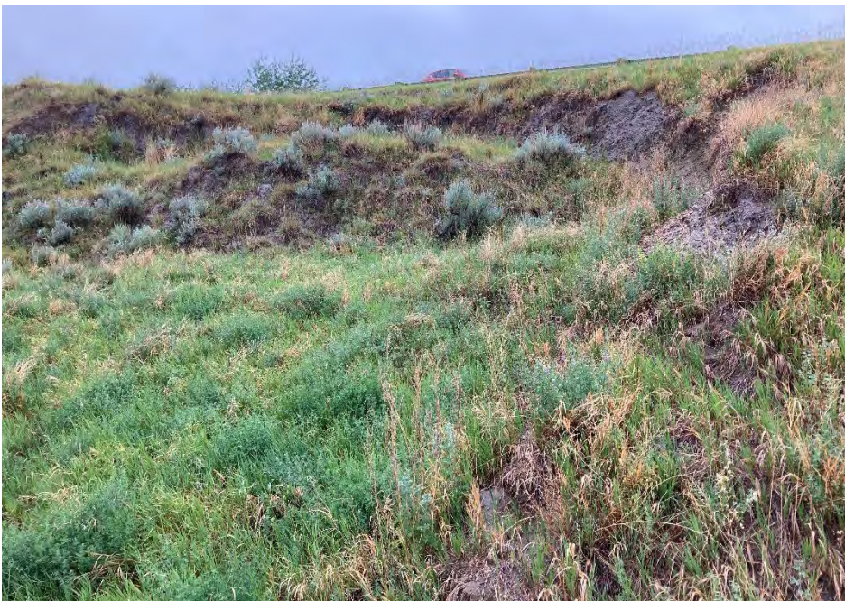
Photo 4 Backscarp of the slide south of Hwy 569. The slide does not appear to have progressed since the inspection in 2020 and appears to be inactive, excluding some minor erosion on the near-vertical backscarp. Photo taken June 24, 2021 facing north.
