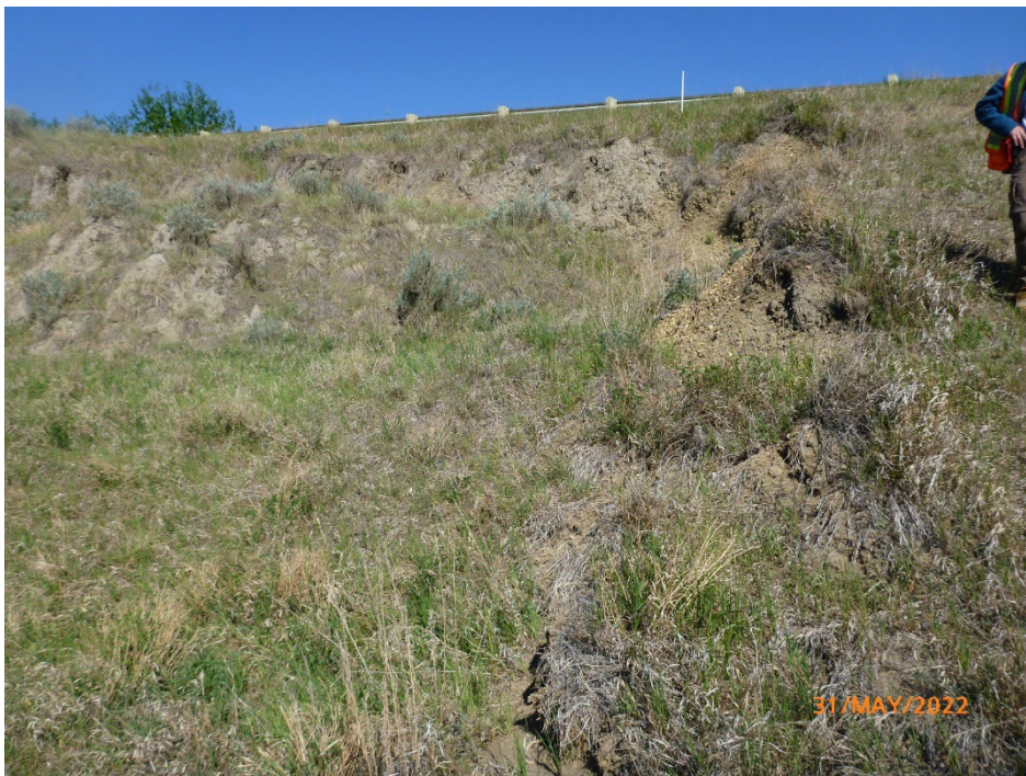
Photo 3 Eastern flank of the slide. Small amount of ongoing erosion occurring on the vertical face where there is no vegetation (Waypoint 167). Photo taken June 14, 2021, facing north.
