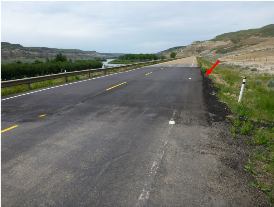
Photo 2 Small sinkhole (0.3 to 0.5 m diameter) along the north edge of pavement at C058-I. Sinkhole is located diagonally from dip in pavement on south side of highway (red circle). Photo taken July 10, 2019 looking southwest.
