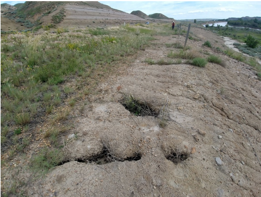
Photo 4 Small sinkholes along the south side of the highway near the fence line at C055-II, west of the culvert outlet (waypoint 22). Photo taken July 10, 2019 looking southeast.
