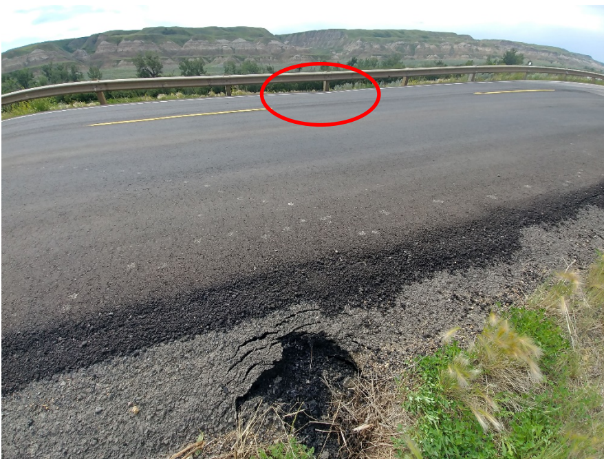
Photo 2 Small sinkhole (0.3 to 0.5 m diameter) along the north edge of pavement at C058-I. Sinkhole is located diagonally from dip in pavement on south side of highway (red circle). Photo taken July 10, 2019 looking southwest.
