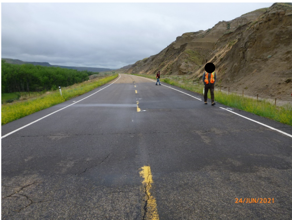
Photo 4 New asphalt patch at C058-II. Settlement in the westbound lane that was holding water from recent precipitation is above the existing culvert. Photo taken June 24, 2021 looking west.
