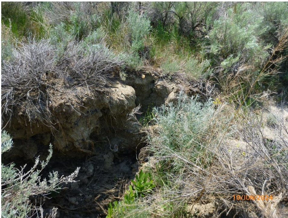
Photo 6 Erosion gully on downstream (south) highway embankment slope. Photo taken June 10, 2025 facing south.
