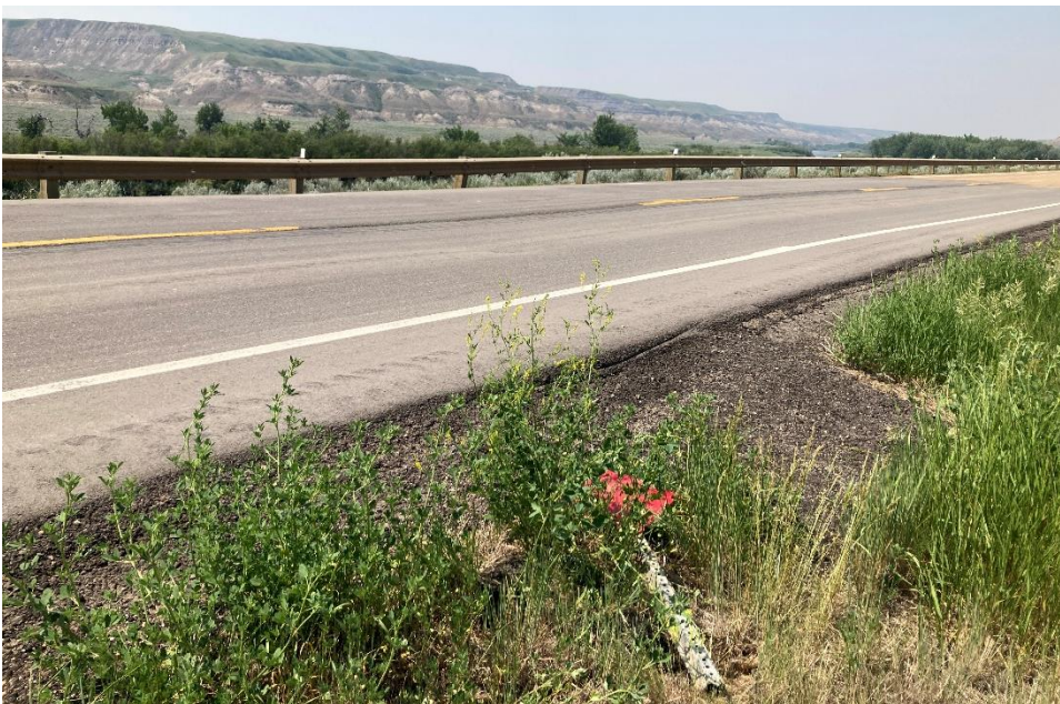
Photo 2 Pavement settlement and sinkhole backfilled with asphalt at the north edge of the highway surface. Red diamond hazard sign lying at the edge of the road. Photo taken June 10, 2025 facing southwest.
