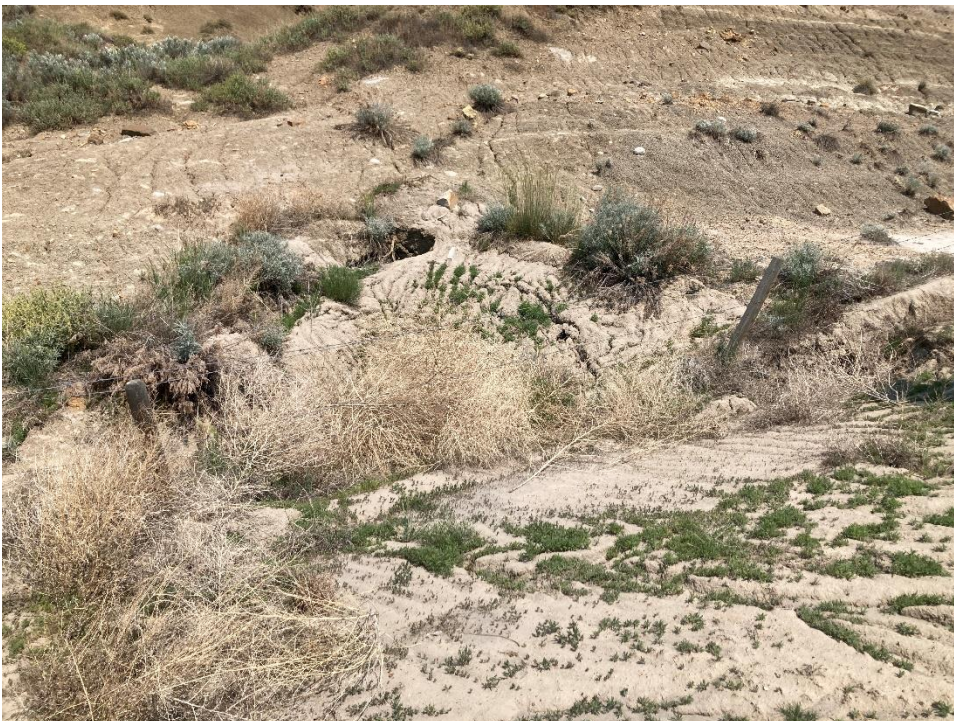
Photo 10 Large sinkhole (approximately 3 m in diameter) in the north (westbound) ditch that is impacting the fence. Photo taken June 10, 2025 facing north.
