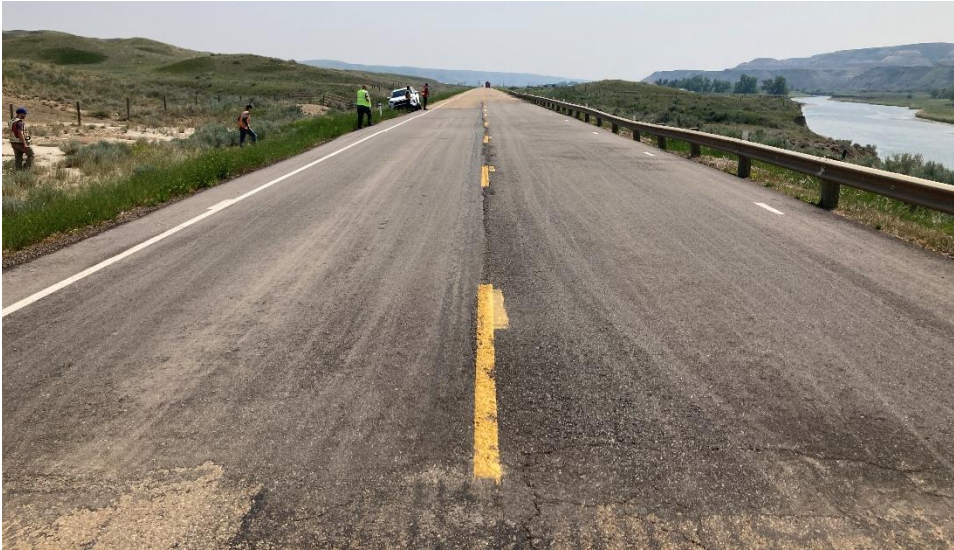
Photo 2 Pavement settlement and sinkhole backfilled with asphalt at the north edge of the highway surface. Red diamond hazard sign lying at the edge of the road. Photo taken June 10, 2025 facing southwest.
