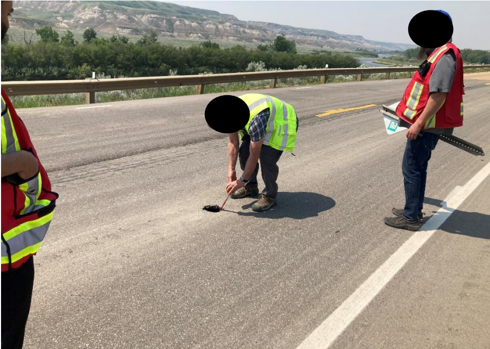
Photo 4 Highway Maintenance Contractor applying spray paint around sinkhole opening. Photo taken June 10, 2025 facing east.
