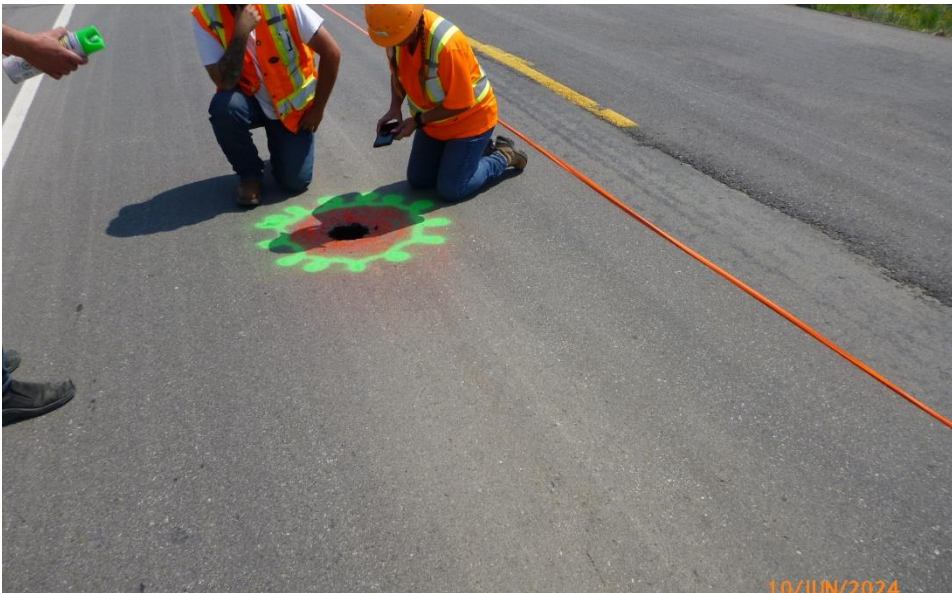
Photo 4 Highway Maintenance Contractor applying spray paint around sinkhole opening. Photo taken June 10, 2025 facing east.
