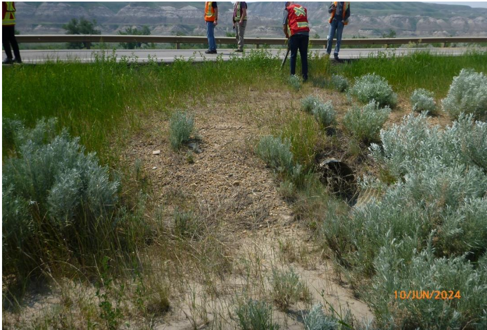
Photo 6 Erosion gully on downstream (south) highway embankment slope. Photo taken June 10, 2025 facing south.
