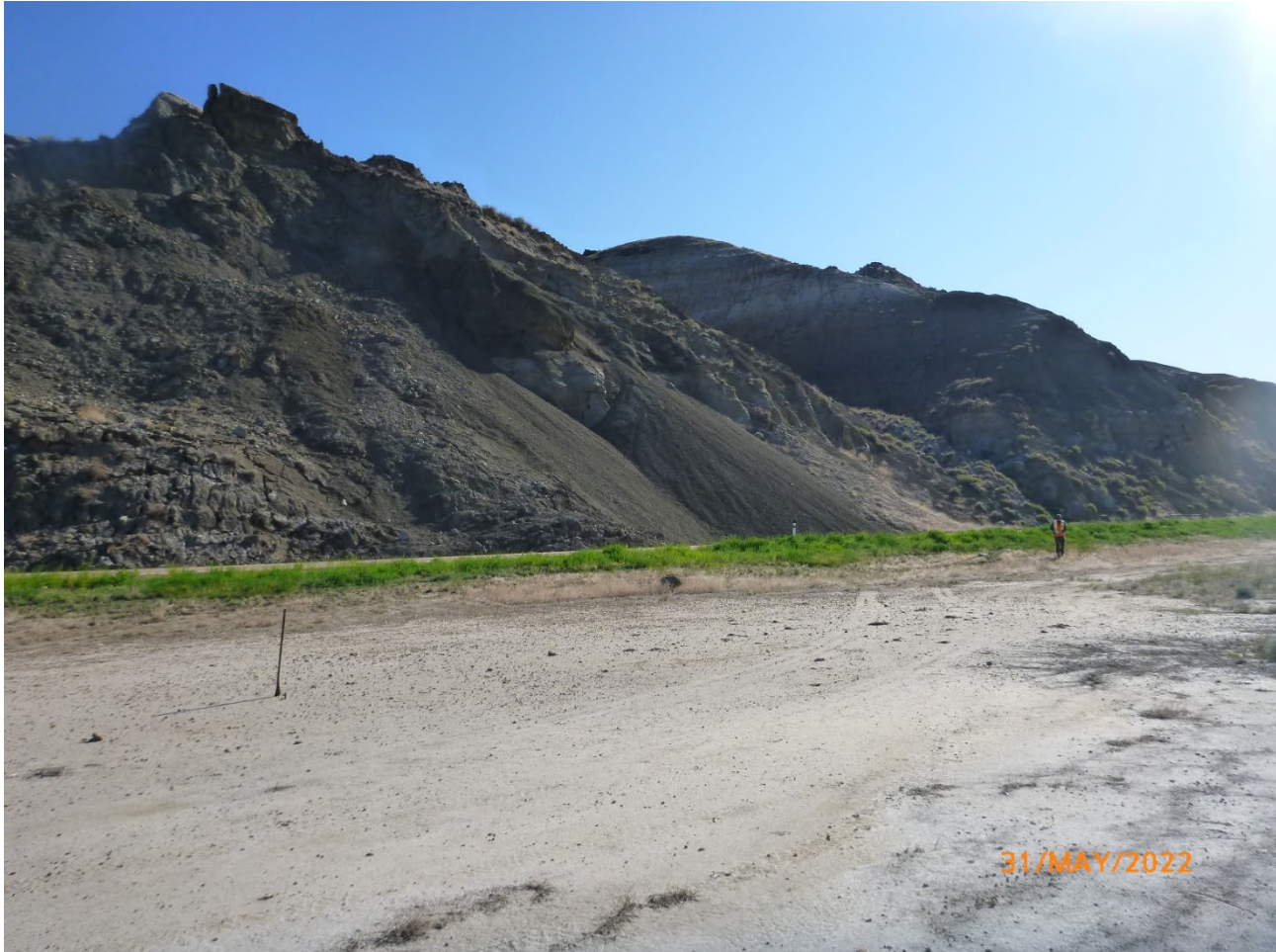
Photo 5 Former natural ground area (ridge) that was excavated for railway and highway construction. Photo taken May 31, 2022, facing northeast.
