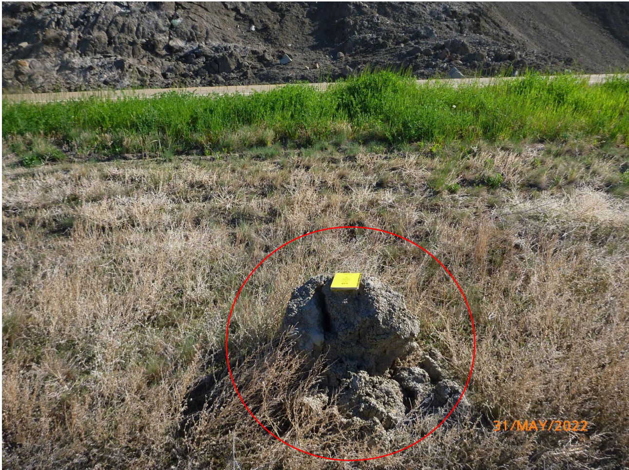
Photo 4 Boulder found across the Highway. Photo taken May 31, 2022, facing north.
