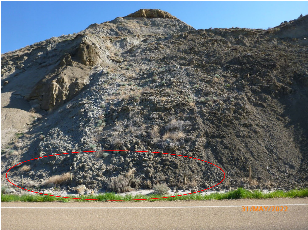
Photo 2 Barbed wire fence covered with talus material along the highway. Photo taken May 31, 2022, facing north.
