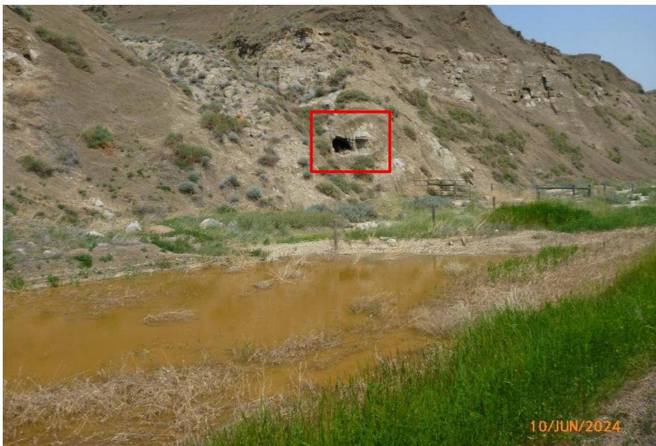
Photo 6 Ponded water along the north (westbound) ditch near the east extent of the site. Sinkhole observed in north slope indicated by red rectangle. Photo taken June 10, 2025 facing northeast.
