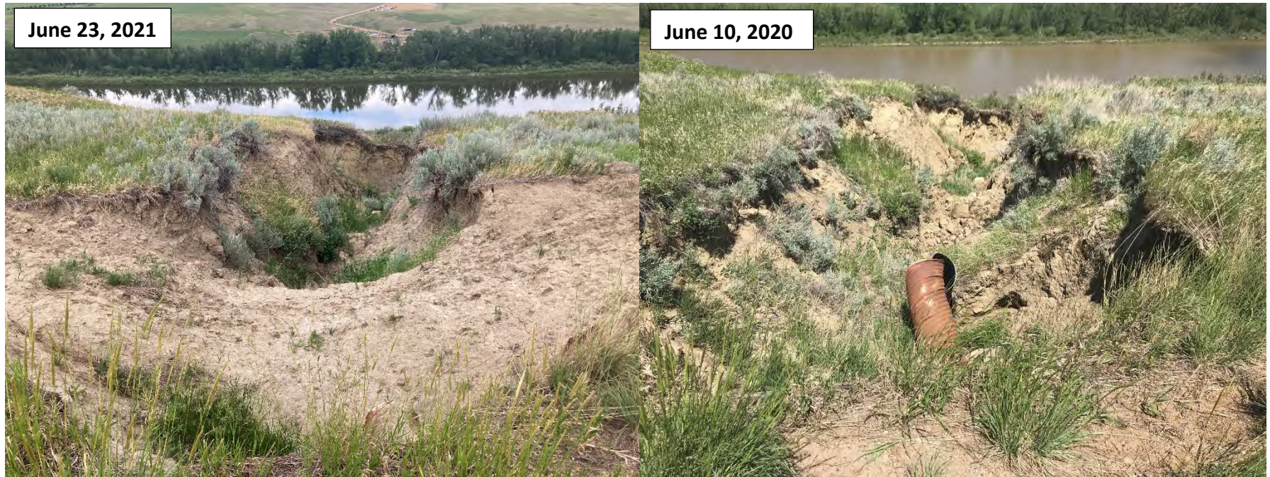
Photo 2 Comparison of the C017-II erosion gully in 2020 and 2021. Gully appears to have been partially backfilled since June 2020, likely due to a traffic accident that resulted in an 18-wheeler truck crashing through the guardrail and into this gully. The inlet of the culvert is locked with soil in the south ditch, but erosion could result in flows discharging into the gully again. The outlet of the 600 mm CSP culvert is detached and hanging. Photos taken looking northeast.
