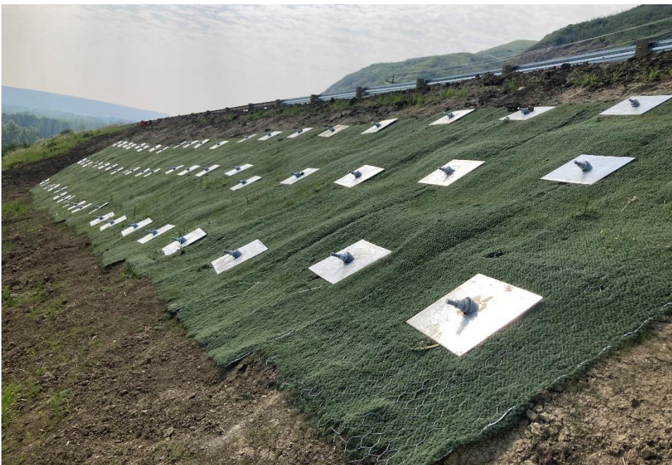
Photo 10 Soil nails, base plates, and slope stabilization product installed in 2025 at C017-1. Photo taken June 10, 2025 facing east.
