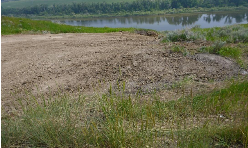
Photo 7 Ditch erosion in south (eastbound) ditch does not appear to have worsened between the 2024 and 2025 inspections. Photo taken June 10, 2025 facing east.
