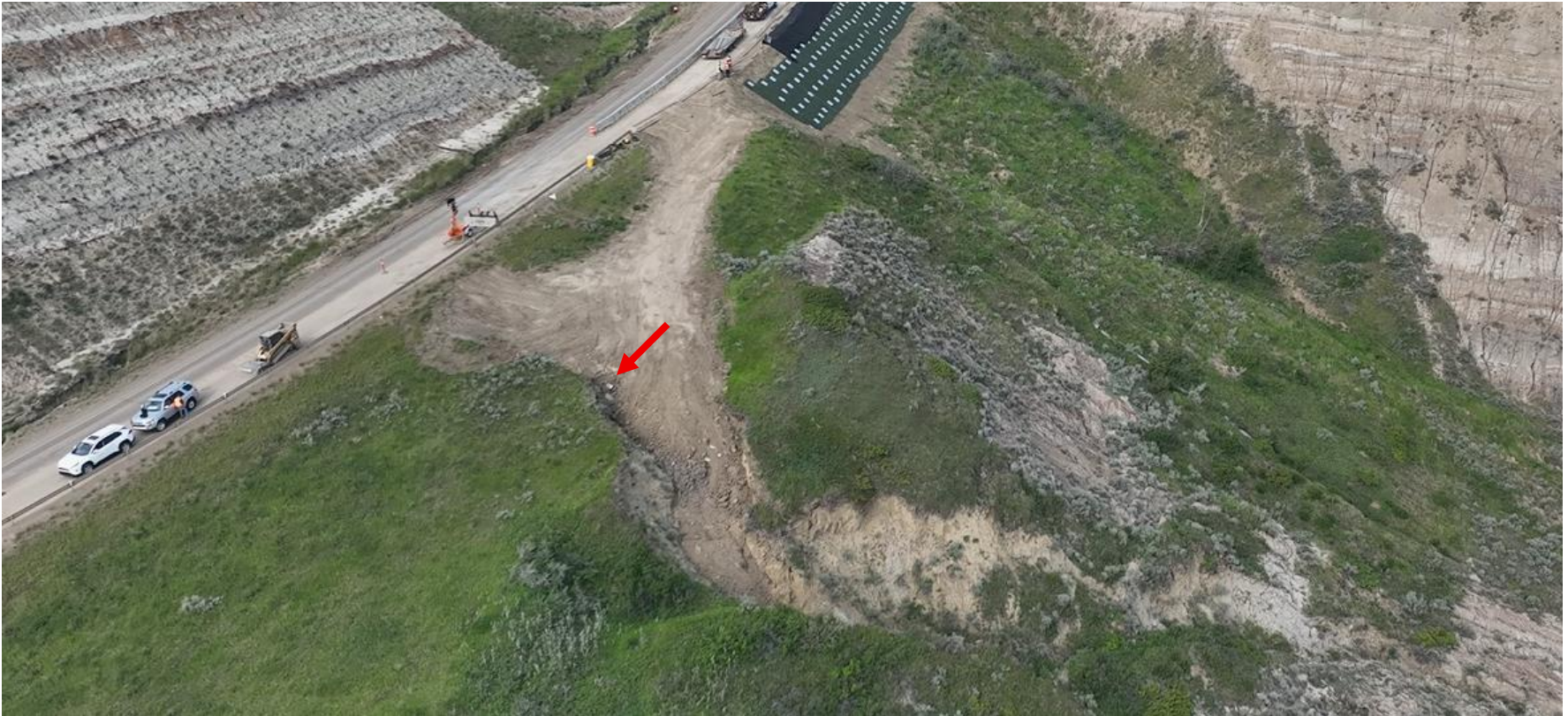
Photo 4 Aerial oblique photo of the C017-2 site. Approximately 20 m of the erosion gully north of the highway backfilled during 2025 construction after extending CSP culvert (outlet indicated by red arrow). Photo taken June 10, 2025 facing west.
