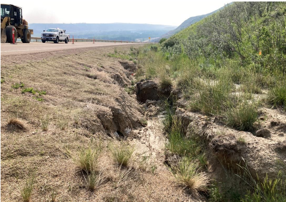
Photo 7 Ditch erosion in south (eastbound) ditch does not appear to have worsened between the 2024 and 2025 inspections. Photo taken June 10, 2025 facing east.
