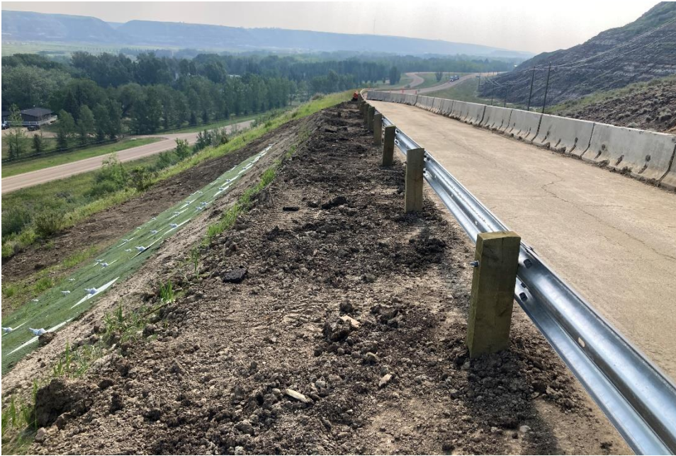
Photo 10 Soil nails, base plates, and slope stabilization product installed in 2025 at C017-1. Photo taken June 10, 2025 facing east.
