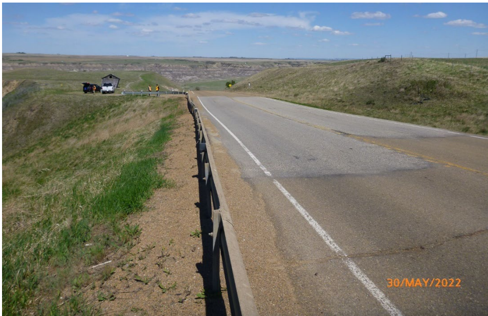
Photo 4 The pavement and guardrail have continued to settle since the 2018 inspection. The guardrail is low due to the regular pavement patching. Photo taken May 30, 2022, facing southeast.
