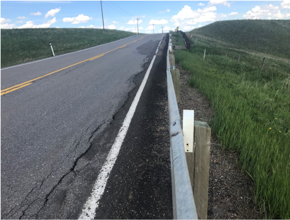
Photo 2 Wooden retaining structure at east end of pile wall has deflected more since the 2019 inspection. Photo taken June 9, 2020 facing north.
