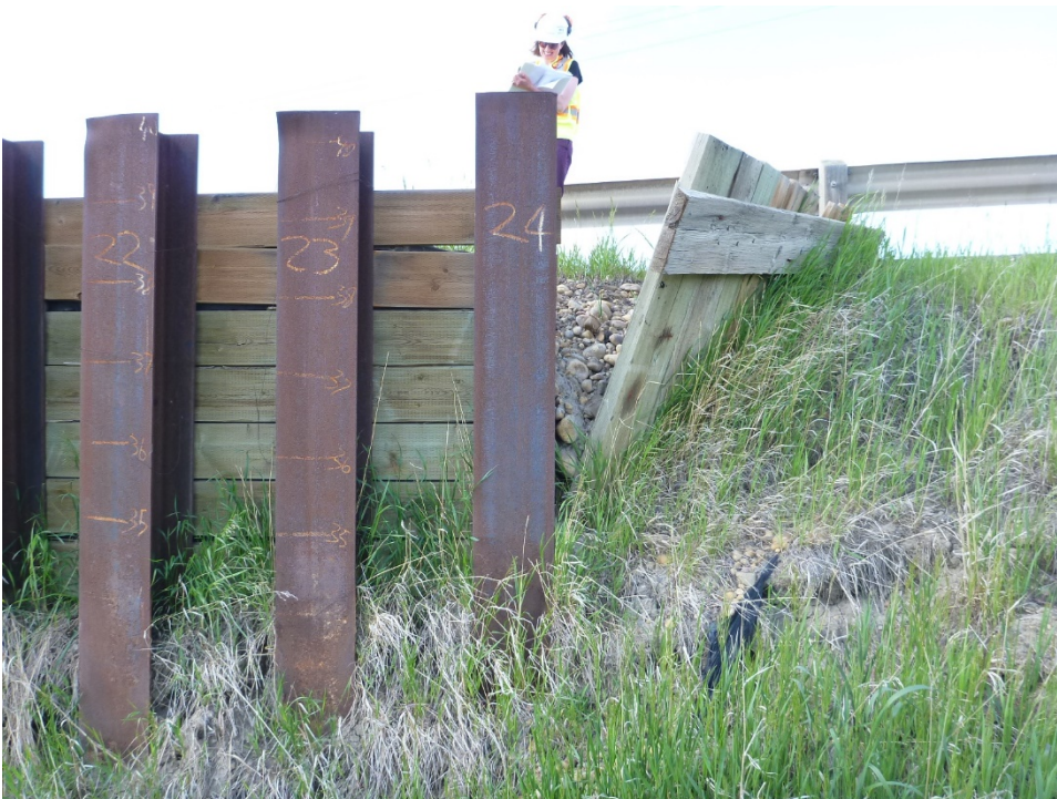
Photo 2 Wooden retaining structure at east end of pile wall has deflected more since the 2019 inspection. Photo taken June 9, 2020 facing north.
