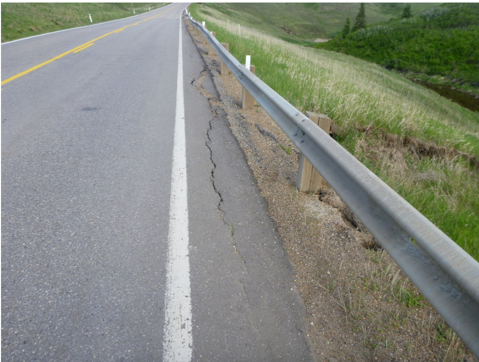
Photo 6 Pavement cracking in eastbound lane above head of slide at C048-III. Cracks appear to have expanded slightly since 2019. Photo taken June 6, 2020 facing east.
