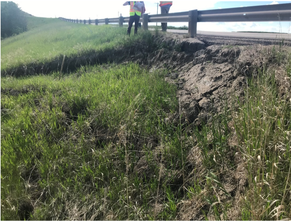
Photo 6 Pavement cracking in eastbound lane above head of slide at C048-III. Cracks appear to have expanded slightly since 2019. Photo taken June 6, 2020 facing east.
