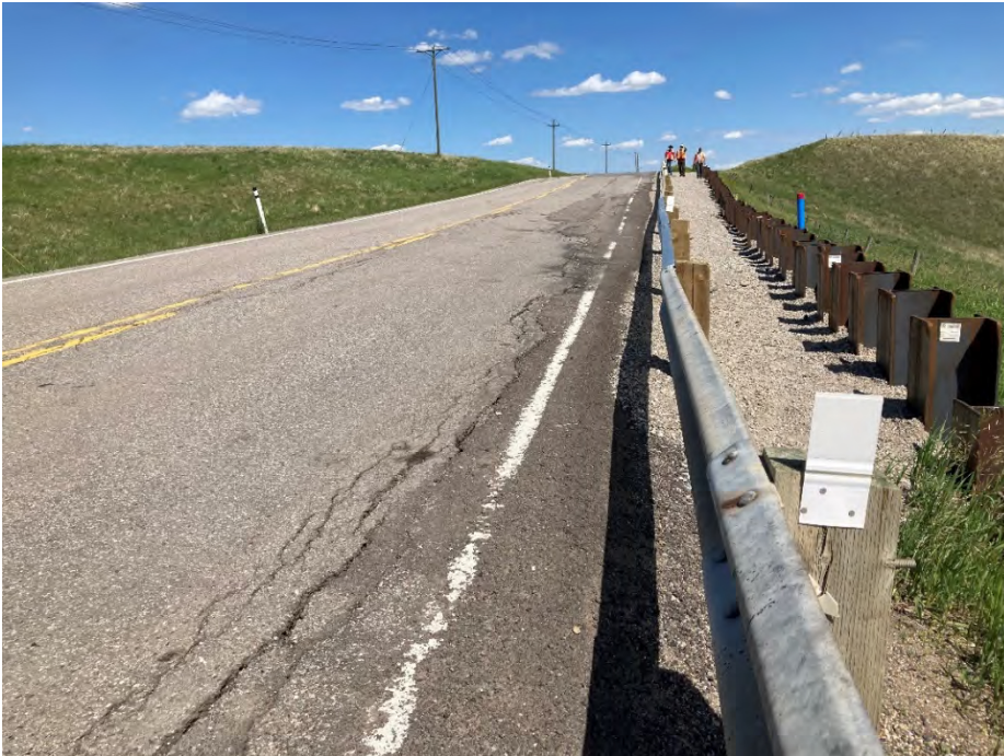
Photo 2 West pile wall extension and wooden planks installed in early-2021. Photo taken June 23, 2021 facing east.
