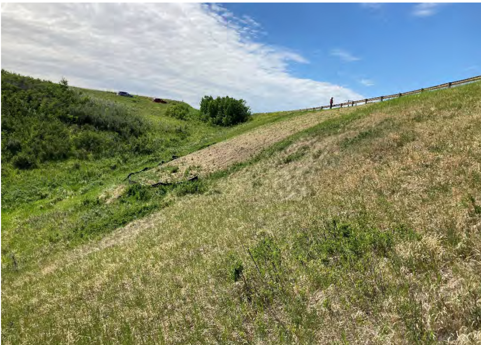
Photo 6 C048-III repair was not graded to match the existing highway embankment slope and there is little to no vegetation (required reseeding). Photo taken June 23, 2021 facing west.
