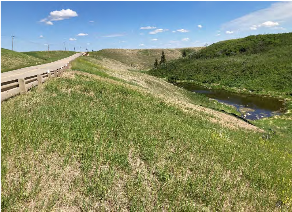
Photo 6 C048-III repair was not graded to match the existing highway embankment slope and there is little to no vegetation (required reseeding). Photo taken June 23, 2021 facing west.
