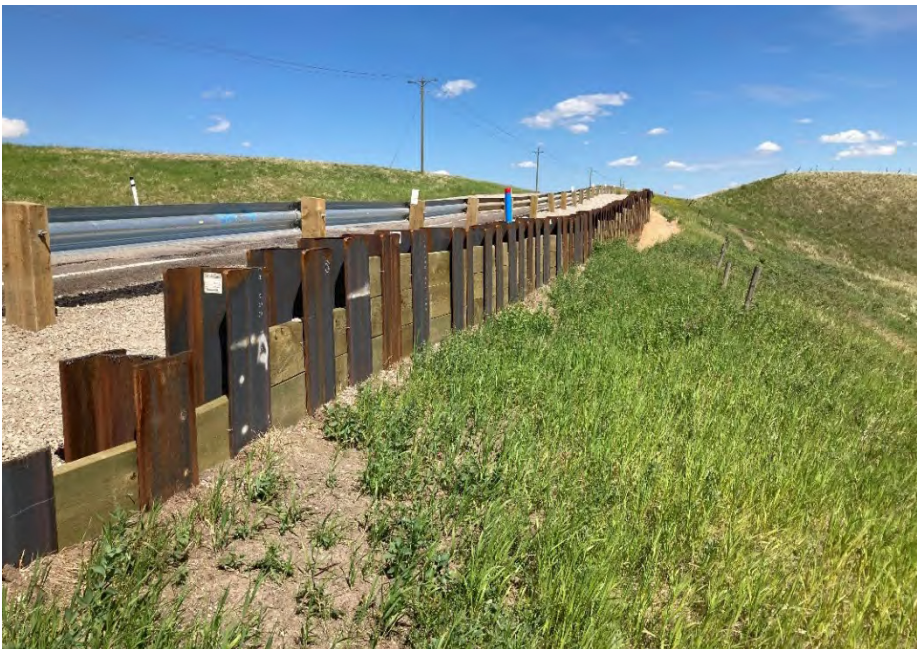
Photo 2 West pile wall extension and wooden planks installed in early-2021. Photo taken June 23, 2021 facing east.
