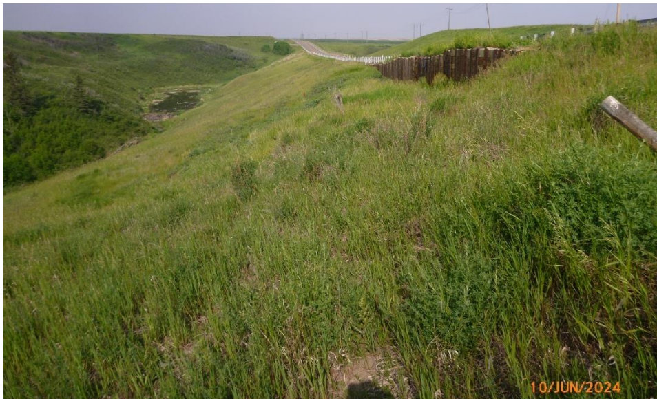
Photo 5 H-pile wall extension, timber lagging, and lower H-pile wall installed in 2021. Downslope of the H-pile walls is well vegetated and in good condition. Photo taken June 10, 2025 facing west.
