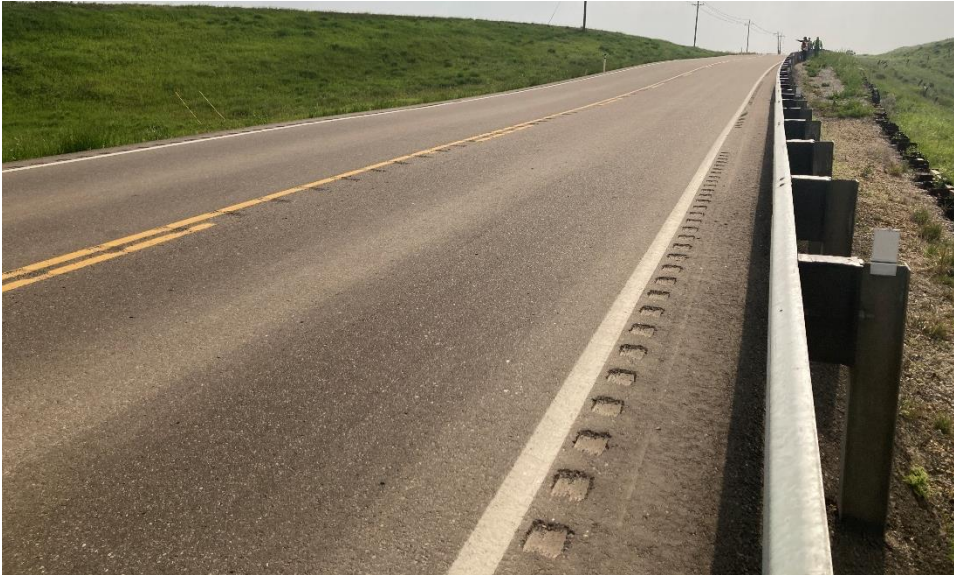
Photo 3 The upper H-pile wall has continued to deflect since the 2023 inspection. Photo taken June 10, 2025 facing east.
