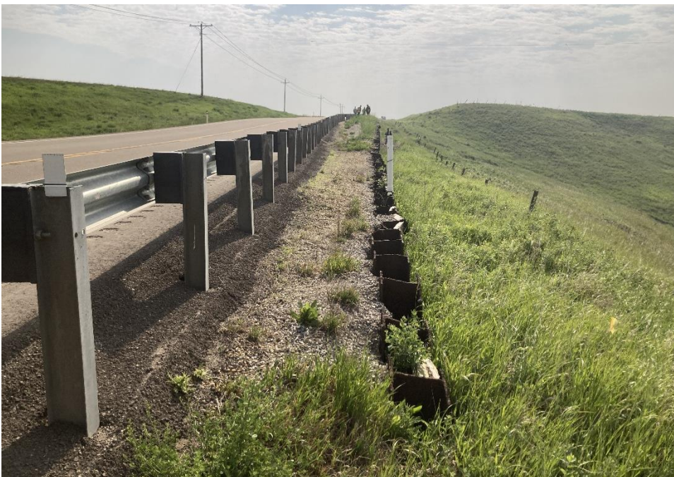
Photo 3 The upper H-pile wall has continued to deflect since the 2023 inspection. Photo taken June 10, 2025 facing east.
