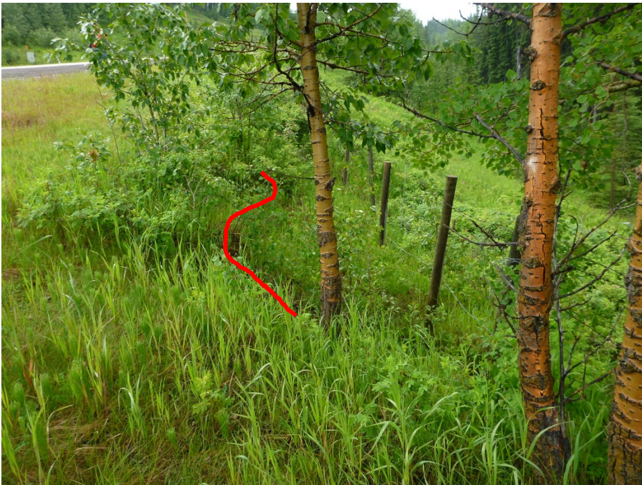
Photo 5 Scarp near fence line in slide area #4 (indicated by red line). Photo taken July 10, 2019 looking southeast.
