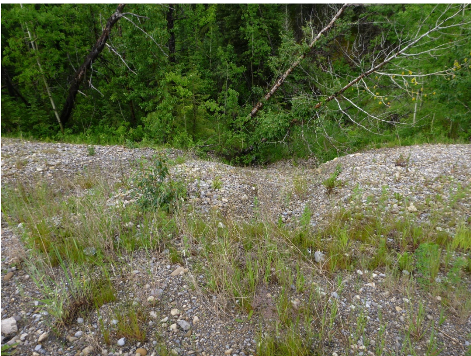
Photo 2 Erosion gullies continue to form in gravel fill below slide area # 2. Photo taken July 10, 2019 looking southwest.
