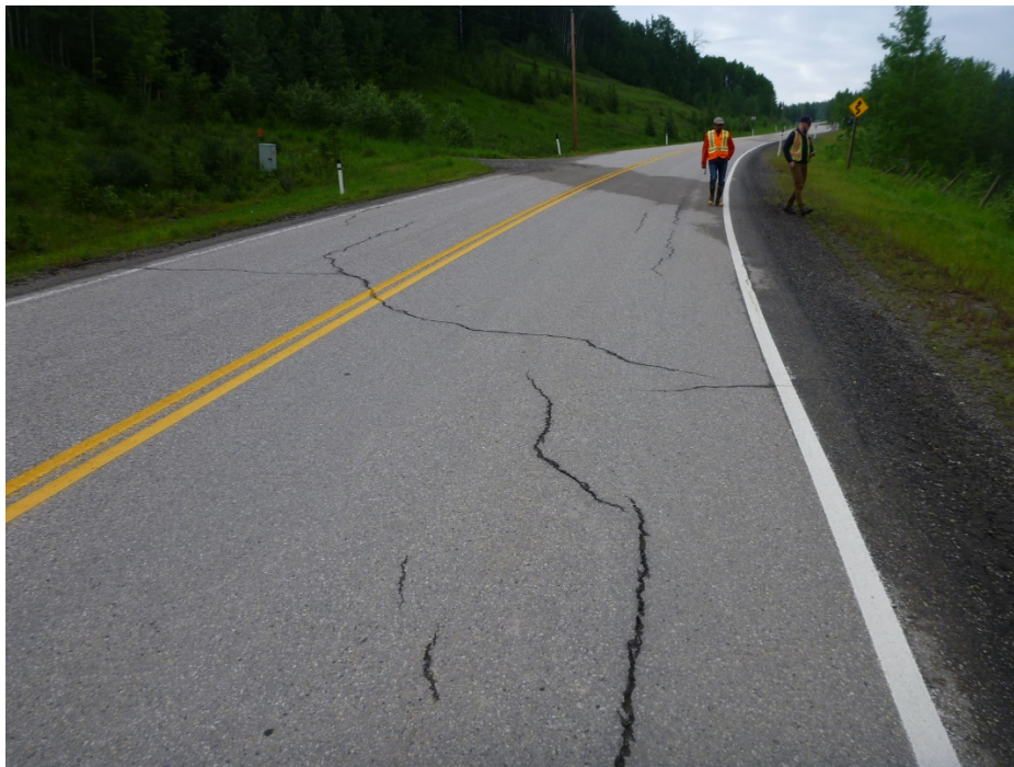
Photo 4 Pavement cracking in eastbound lane in slide area #4. Photo taken July 10, 2019 looking southeast.
