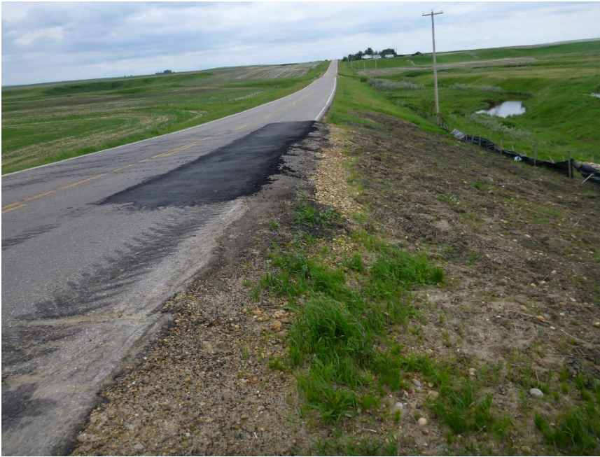
Photo 2 The fence is tilted and the silt fence is damaged. Photo taken June 13, 2017 looking west.
