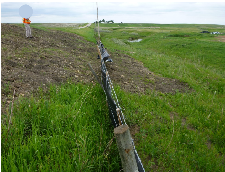
Photo 2 The fence is tilted and the silt fence is damaged. Photo taken June 13, 2017 looking west.
