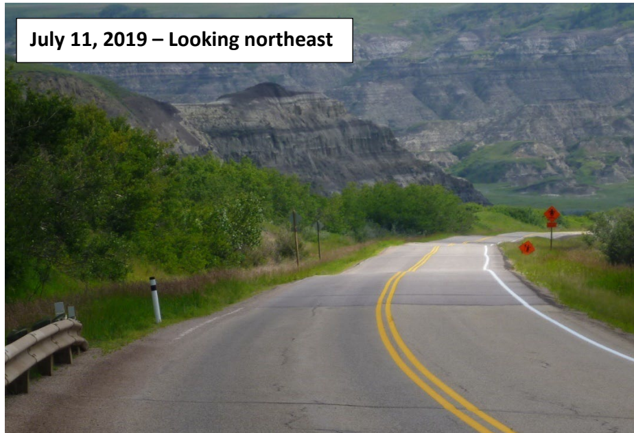
Photo 4 Photo showing the pavement dips at the C065-II site in 2018 and 2019 from opposite directions. Pavement dips appear to have worsened since 2018.
