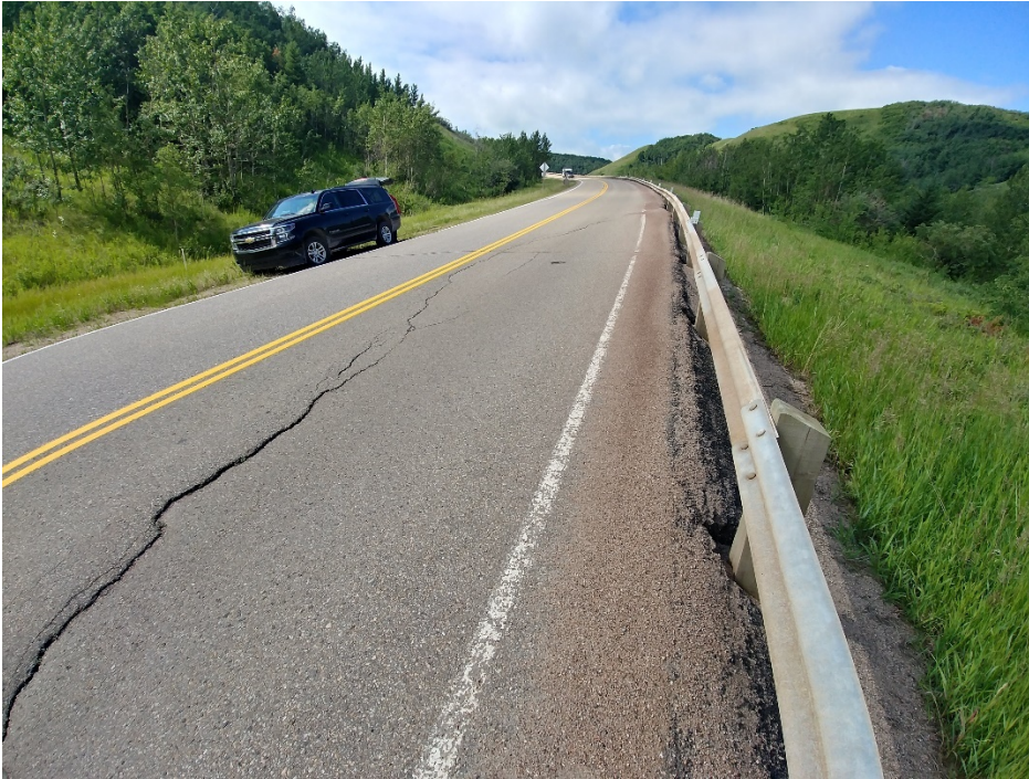
Photo 7 View of the highway surface at the C065-IV site. Pavement deflection appears to have increased slightly since 2018 inspection. Photo taken July 11, 2019 looking southwest.
