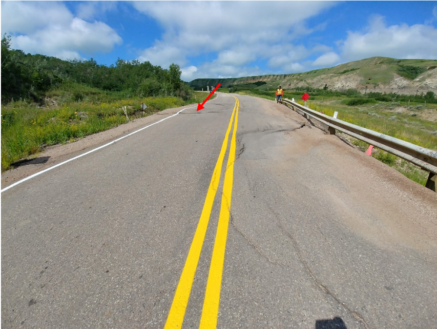
Photo 2 Close-up view showing the severity of pavement deflection in the westbound lane at C065-I. Pavement has deflected up to 4". Photo taken July 11, 2019 looking east.
