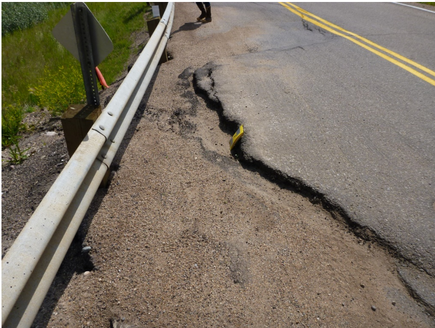
Photo 2 Close-up view showing the severity of pavement deflection in the westbound lane at C065-I. Pavement has deflected up to 4". Photo taken July 11, 2019 looking east.
