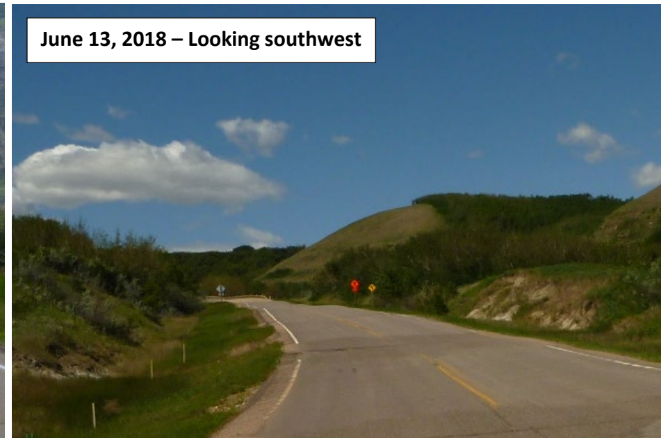
Photo 4 Photo showing the pavement dips at the C065-II site in 2018 and 2019 from opposite directions. Pavement dips appear to have worsened since 2018.
