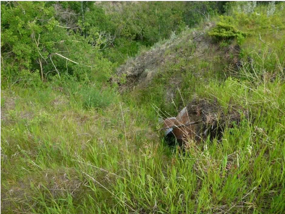
Photo 6 Erosion gully below the undermined culvert outlet at C065-III appears to have increased in size since 2018. Photo taken July 11, 2019 looking north.
