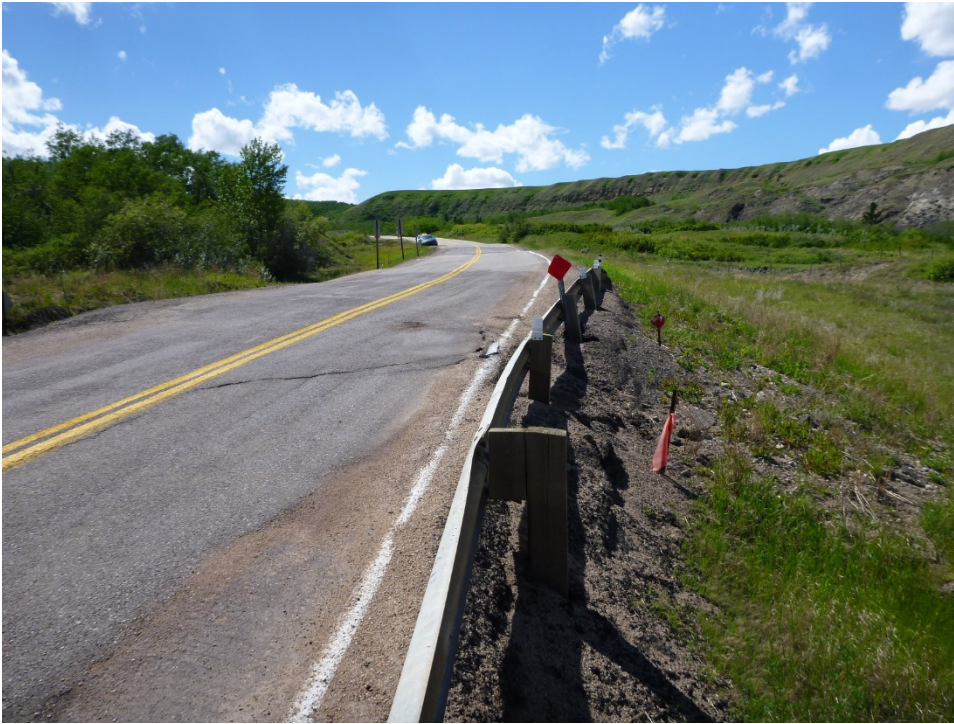
Photo 2 Wooden guardrail posts have deflected horizontally due to the movement of the highway. Photograph taken June 9, 2020 facing north.
