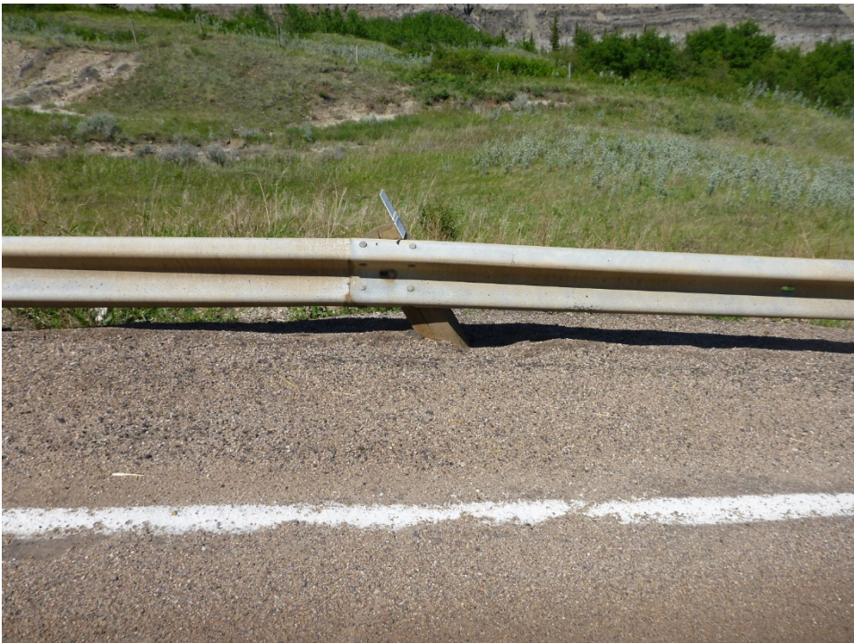
Photo 2 Wooden guardrail posts have deflected horizontally due to the movement of the highway. Photograph taken June 9, 2020 facing north.
