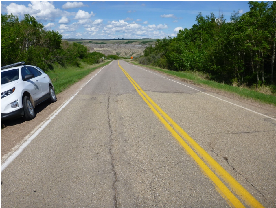
Photo 6 View of the highway surface at the C065-IV site. Pavement deflection appears to have increased slightly since 2019 inspection. Photo taken June 9, 2020 facing east.
