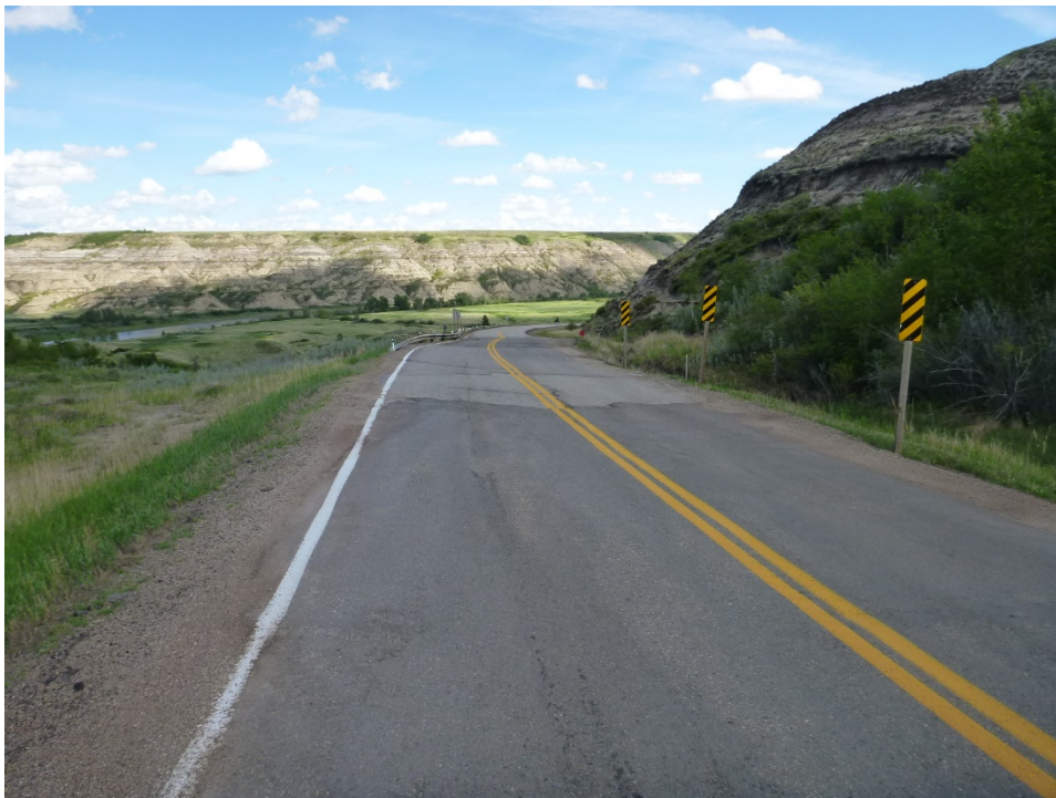
Photo 4 Toe roll in pavement (red circle) caused by heavy trucks braking at they approach the C065-I site. Photo taken June 9, 2020 facing east.
