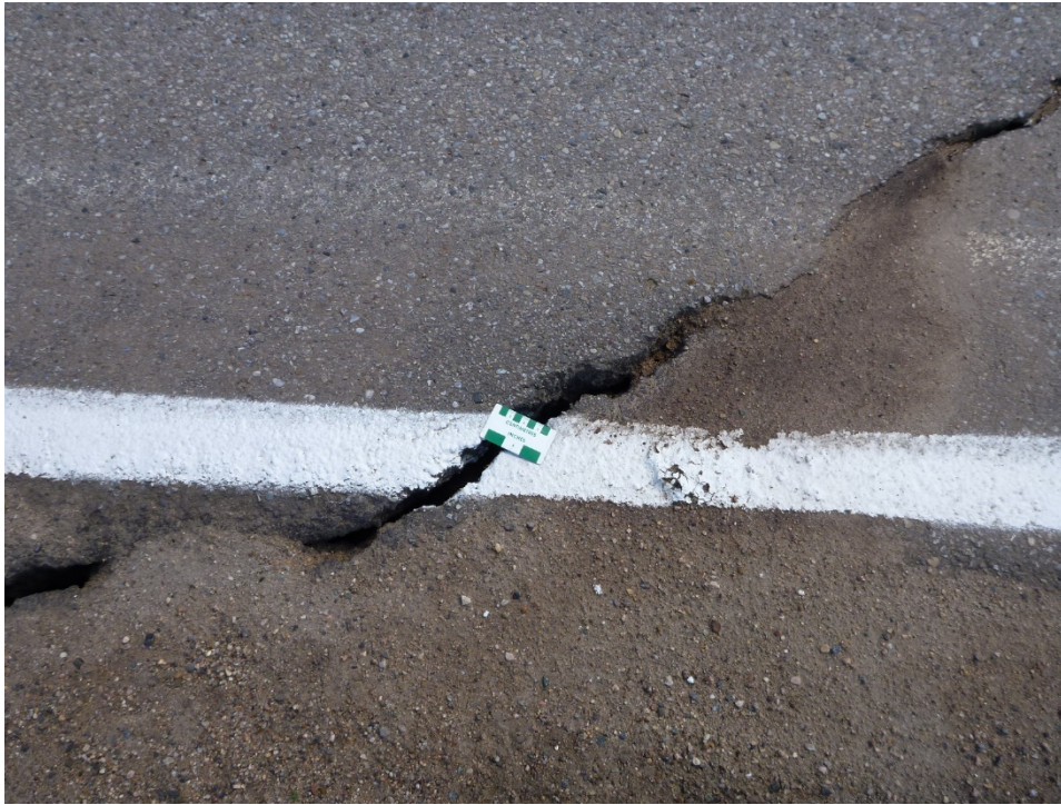
Photo 4 Toe roll in pavement (red circle) caused by heavy trucks braking at they approach the C065-I site. Photo taken June 9, 2020 facing east.
