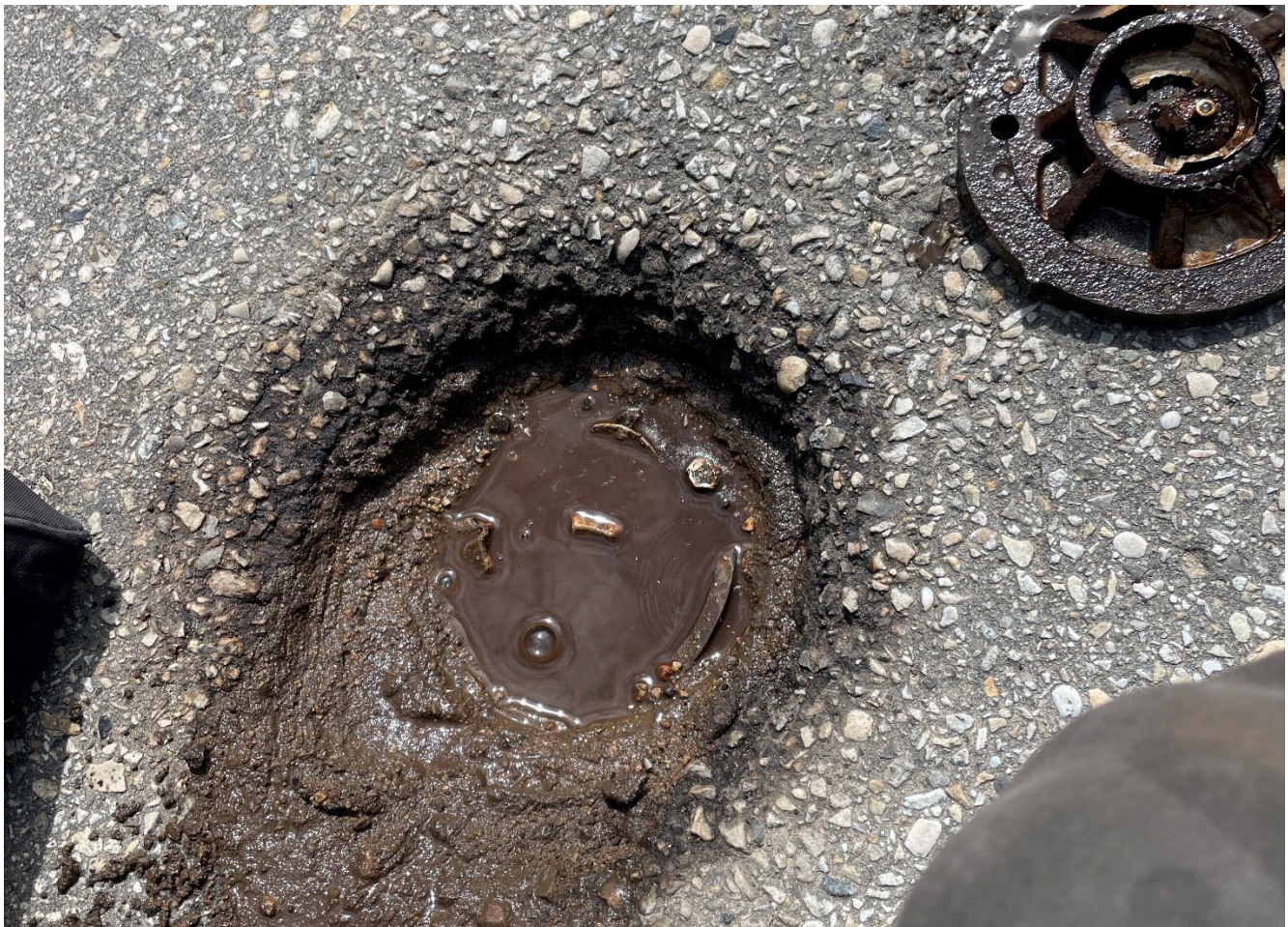
Photo 3.1 Sand and turbid water inside the flush-mounted headbox at the C065-3 subsite.
