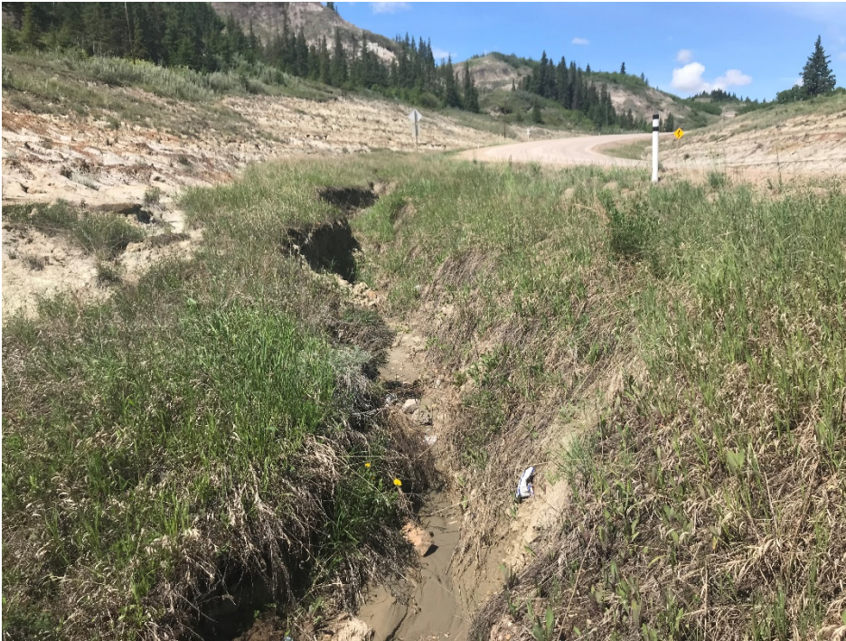
Photo 3 The outlet of the 1200 mm diameter CSP to the west of the bridge. Photo taken June 9, 2020 looking west.
