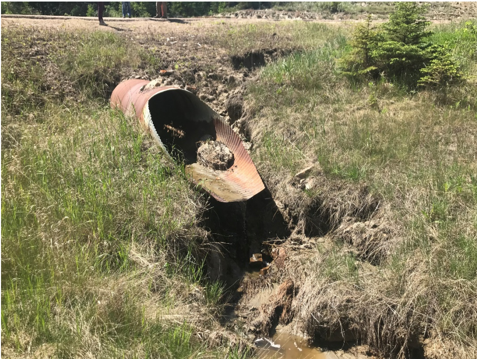
Photo 3 The outlet of the 1200 mm diameter CSP to the west of the bridge. Photo taken June 9, 2020 looking west.
