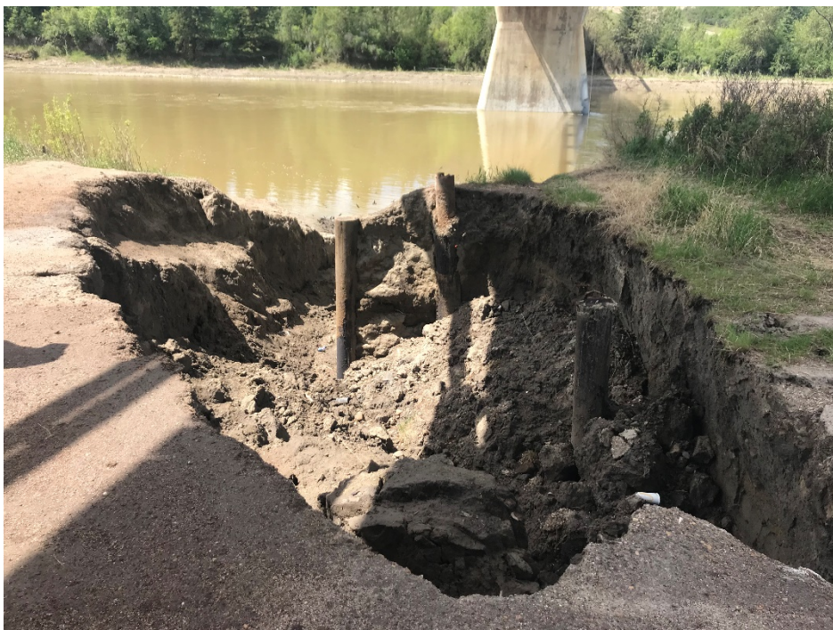
Photo 6 Erosion gully below east bridge abutment continues to expand. Photo taken June 9, 2020 looking west.
