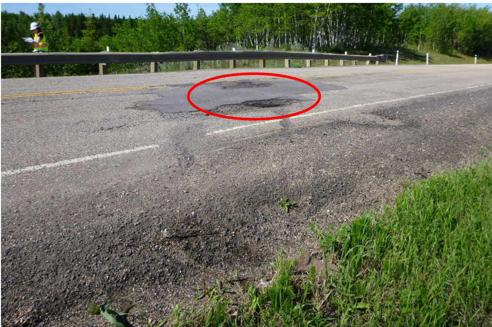
Photo 2 Photo showing the condition of pavement above the slide area. Condition of pavement in the westbound lane (red ellipse) has worsened since the 2019 inspection. Photo taken June 9, 2020 looking southwest.
