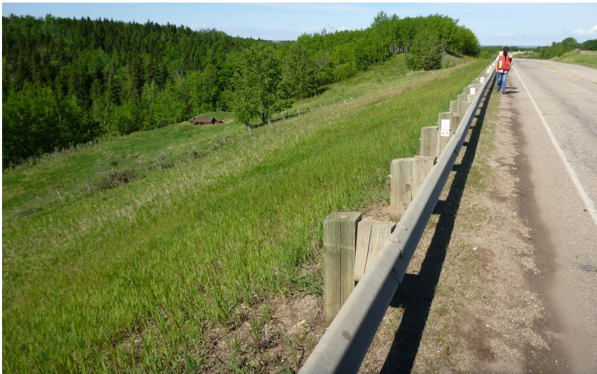
Photo 4 Slope below highway showing no signs of deformation or slope movement since 2019 inspection. Photo taken June 9, 2020 facing west.
