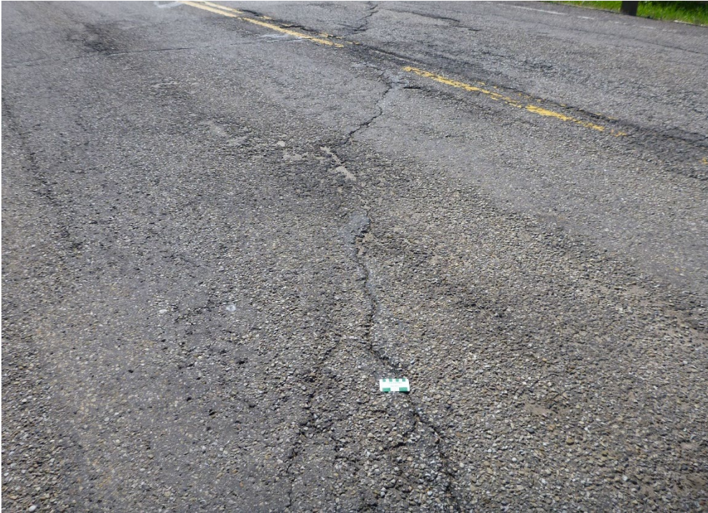
Photo 2 Photo showing the condition of pavement above the slide area. Condition of pavement in the westbound lane (red ellipse) has worsened since the 2019 inspection. Photo taken June 9, 2020 looking southwest.
