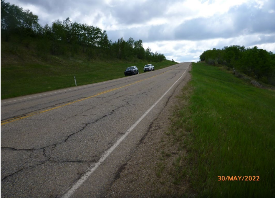
Photo 6 Pavement cracking and settlement above the C008 slide. Photo taken May 30, 2022, facing southeast.
