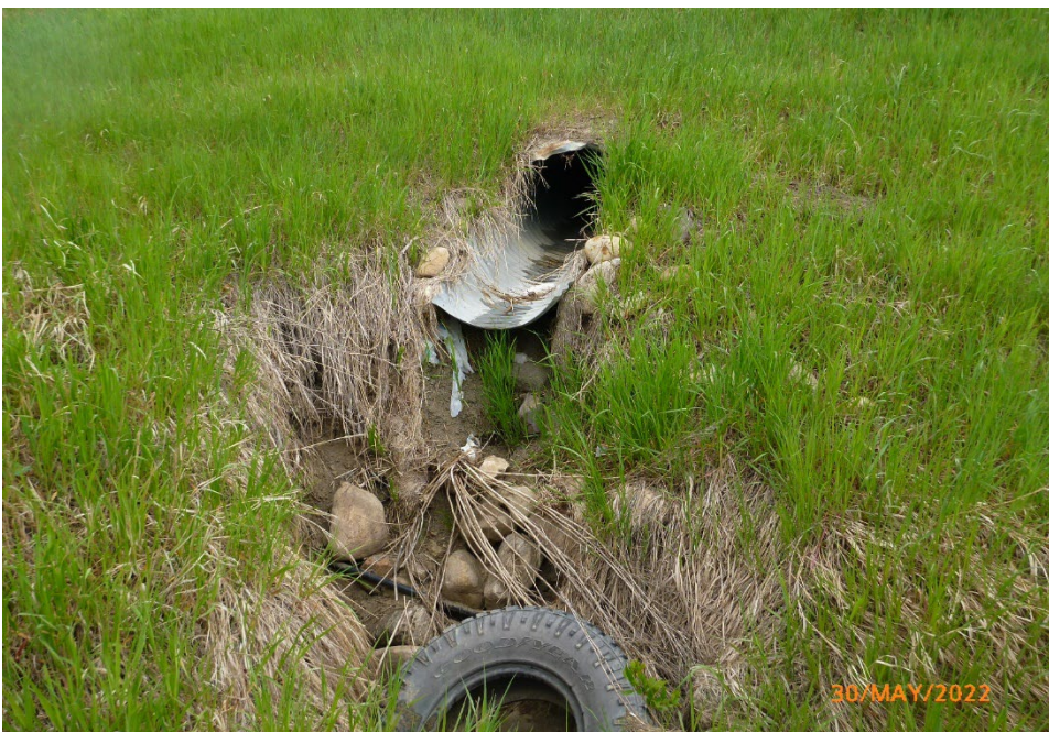
Photo 4 An erosion gully has formed at the CSP culvert underlying Hwy 597 (WP 142) between the 2020 and 2022 inspections. Photo taken May 31, 2022, facing north.
