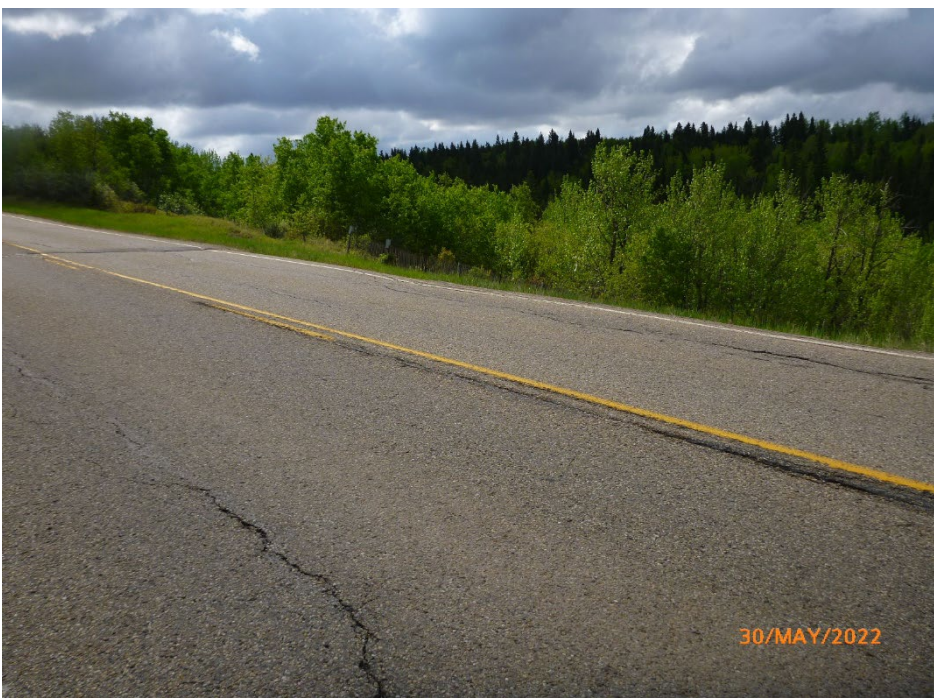
Photo 6 Pavement cracking and settlement above the C008 slide. Photo taken May 30, 2022, facing southeast.
