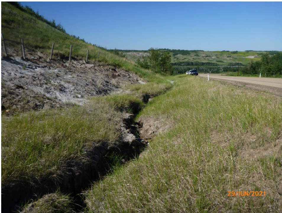
Photo 6 Erosion gully in the north (westbound) ditch is retrogressing towards Hwy 609. Photo taken June 29, 2021 facing east.
