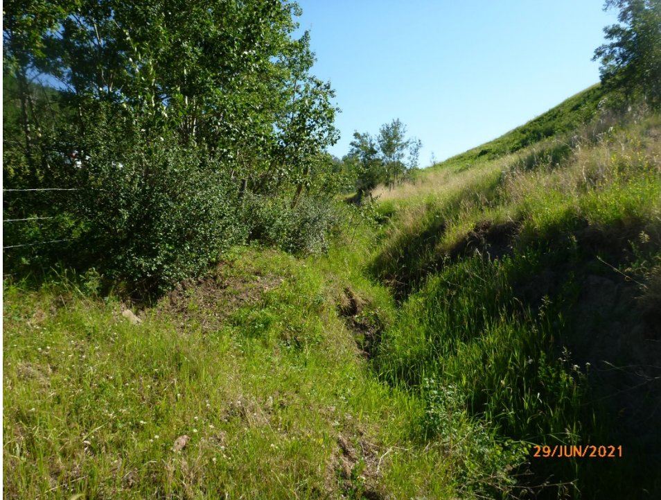
Photo 4 The erosion gully downstream of the north (westbound) ditch, downstream of the CSP culvert outlet has worsened since the 2020 call-out site visit. Photo taken June 29, 2021 facing north.
