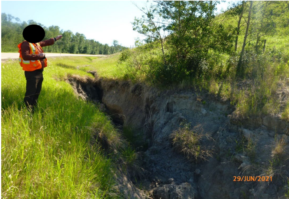
Photo 6 Erosion gully in the north (westbound) ditch is retrogressing towards Hwy 609. Photo taken June 29, 2021 facing east.
