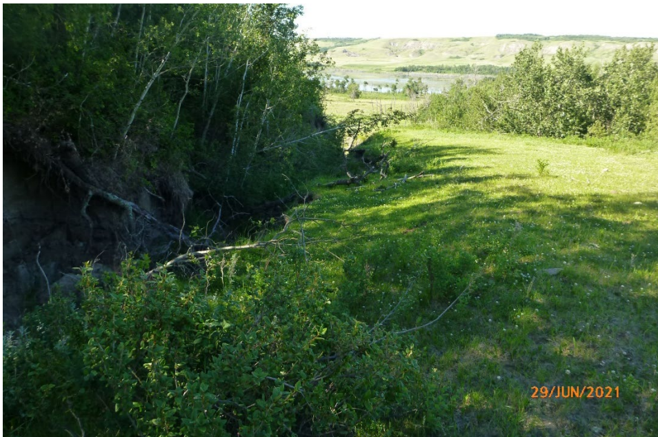
Photo 4 The erosion gully downstream of the north (westbound) ditch, downstream of the CSP culvert outlet has worsened since the 2020 call-out site visit. Photo taken June 29, 2021 facing north.
