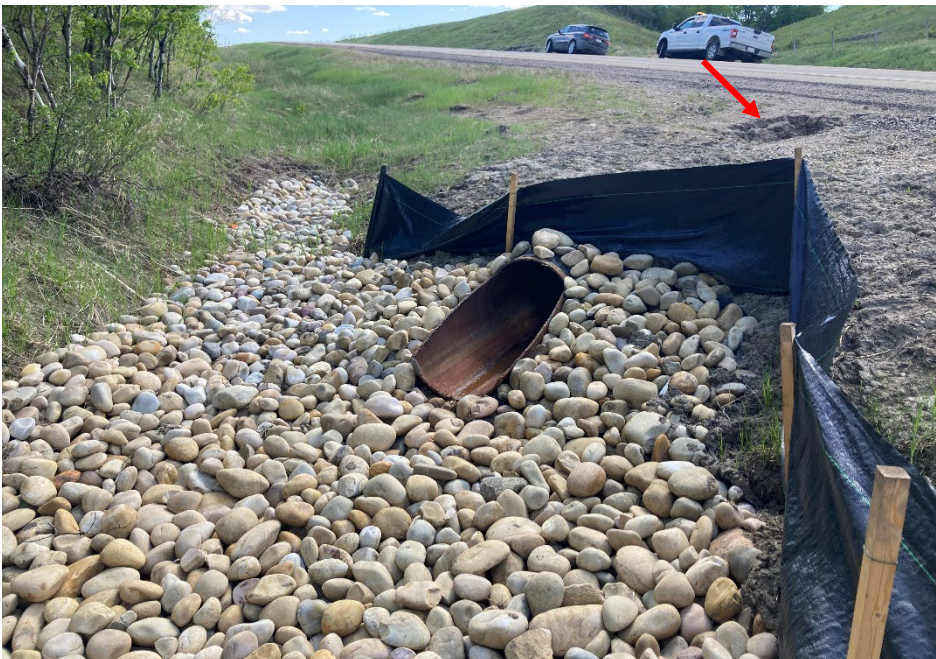
Photo 8 The outlet of the culvert underlying Hwy 56:16. A possible sinkhole was observed near the east (northbound) pavement (indicated by red arrow). Photo taken May 31, 2022, facing south-southwest.
