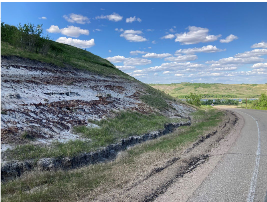
Photo 6 Ditch erosion in the north (westbound) ditch along bedrock outcrop (toe of the cutslope). Photo taken May 31, 2022, facing northeast.
