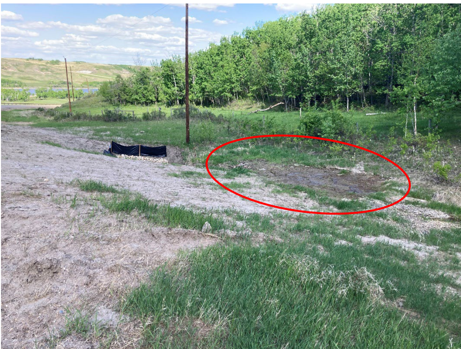
Photo 4 A soft and wet area was observed in the south (eastbound) ditch upstream of the culvert inlet (indicated by red circle). Photo taken May 21, 2022, facing east-southeast.
