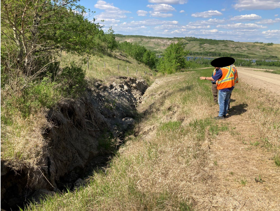
Photo 6 Ditch erosion in the north (westbound) ditch along bedrock outcrop (toe of the cutslope). Photo taken May 31, 2022, facing northeast.
