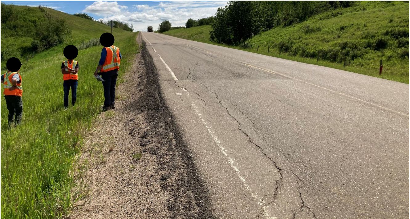
Photo 2 Asphalt settlement in the westbound lane. Photo taken June 24, 2020 facing west.
