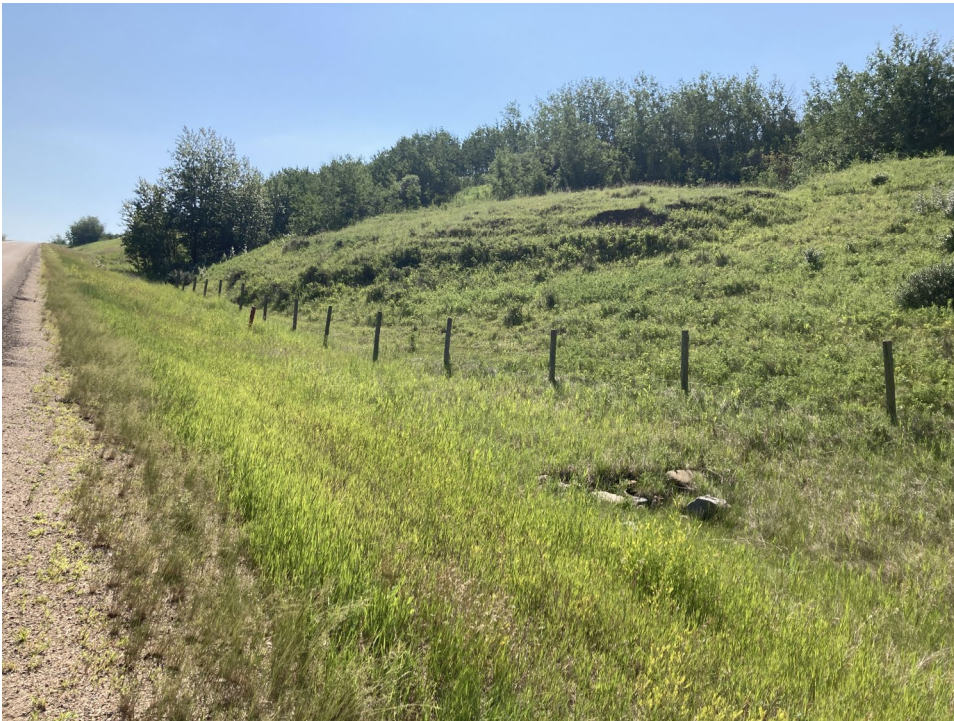
Photo 4 The slide on the cutslope on the south side of Hwy 619:06 appears similar to during the 2021 inspection. Photo taken June 28, 2023, facing southeast.
