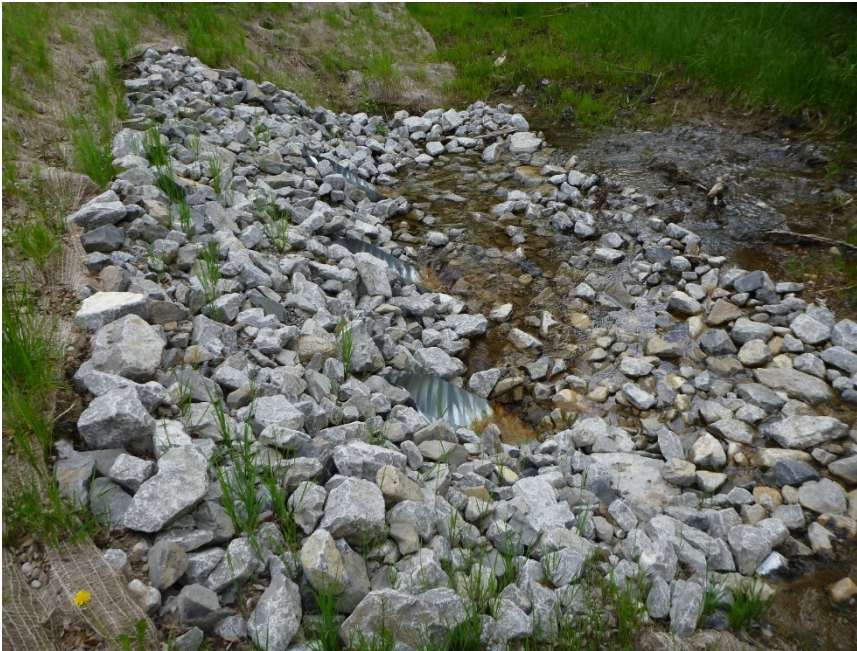
Photo 2 The inlet of the 1000-mm culverts (BF83184) that were installed at the C037 – II site in June 2016. Vegetation is growing through erosion control cloth that was placed around the culverts in June 2016. Photo taken June 12, 2017 looking northeast.
