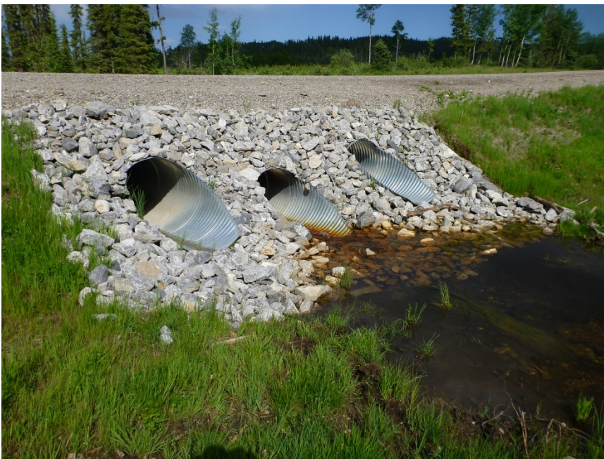
Photo 2 The inlet of the 1000-mm culverts (BF83184) that were installed at the C037 – II site in June 2016. Vegetation is growing through erosion control cloth that was placed around the culverts in June 2016. Photo taken June 12, 2017 looking northeast.
