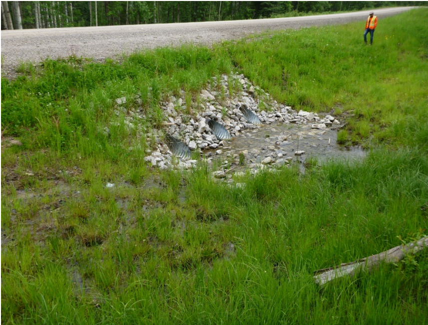
Photo 2 The inlet of the 1000-mm culverts (BF83184) installed at the C037 – II site . Vegetation is growing through riprap placed around culverts. Photo taken July 9, 2019 looking northeast.
