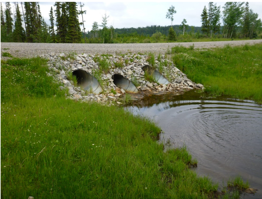
Photo 2 The inlet of the 1000-mm culverts (BF83184) installed at the C037 – II site . Vegetation is growing through riprap placed around culverts. Photo taken July 9, 2019 looking northeast.
