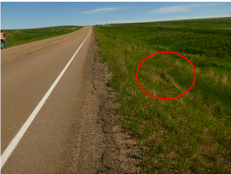
Photo 2 Photo showing evidence of ground cracking extending to the north as indicated by the red circle (waypoint 703) of the backscarp (1-2m) Photo taken June 13, 2018 looking north.
