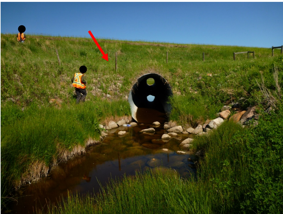
Photo 4 Culvert (BF73719) at the toe of the slide appears to be in good condition. Toe roll of the slide remains above the crown of the culvert as indicated by the red arrow (waypoint 705). Photo taken June 13, 2018 looking northeast.
