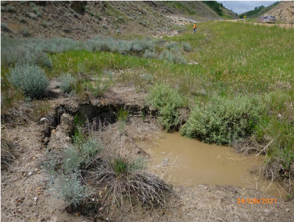
Photo 8 Sinkhole observed approximately mid-slope on the east highway embankment slope. The sinkhole was approximately 3 m wide and 3.5 m long (depth not measured). Photo taken June 24, 2021 facing north.
