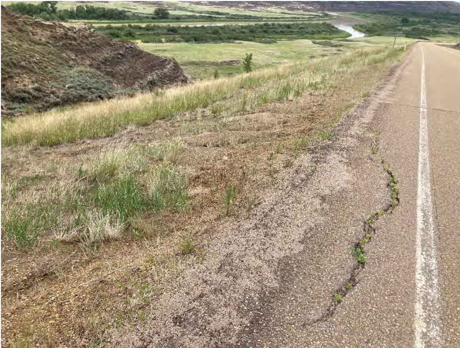
Photo 6 Slope failure triggered by gully erosion at the toe of the slope north of Hwy 837 doesn't appear to have changed since the 2020 inspection. Photo taken June 24, 2021 facing southeast.
