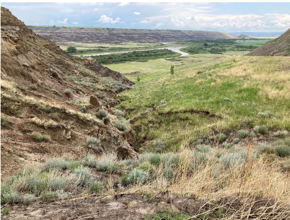
Photo 6 Slope failure triggered by gully erosion at the toe of the slope north of Hwy 837 doesn't appear to have changed since the 2020 inspection. Photo taken June 24, 2021 facing southeast.
