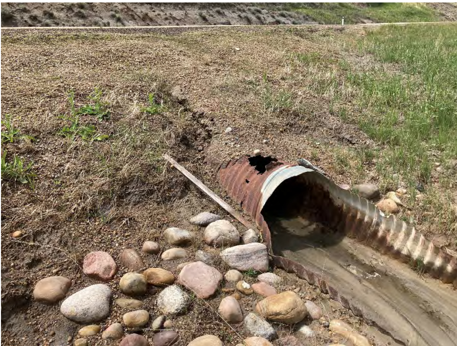
Photo 4 The CSP culvert underlying Hwy 837 (oriented east to west) is corroding, and appears to be in worse condition since the 2020 inspection. Photo taken June 24, 2021 facing northwest.
