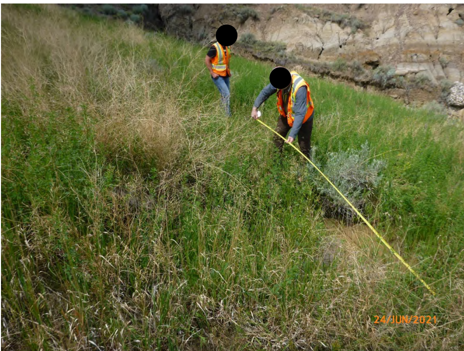
Photo 8 Sinkhole observed approximately mid-slope on the east highway embankment slope. The sinkhole was approximately 3 m wide and 3.5 m long (depth not measured). Photo taken June 24, 2021 facing north.
