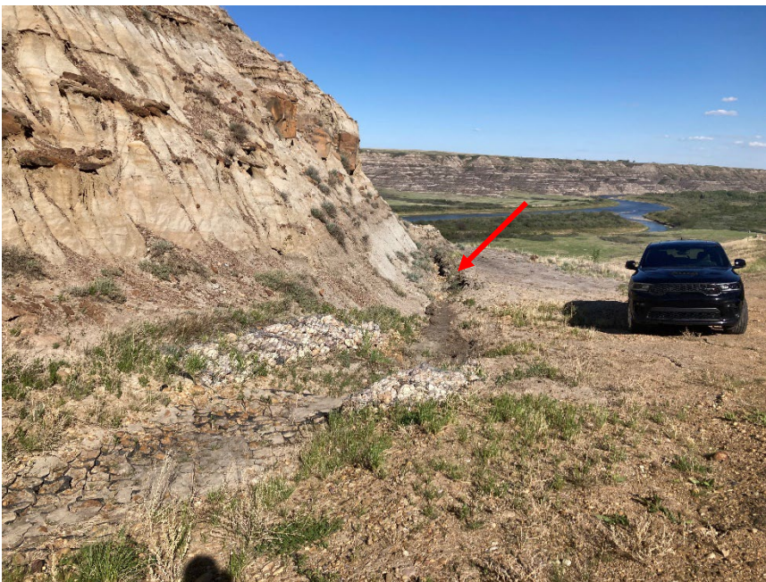
Photo 2 Gully erosion downstream of the gabion baskets (indicated by red arrow) is in similar condition since the 2021 inspection. Photo taken May 30, 2022, facing southeast.
