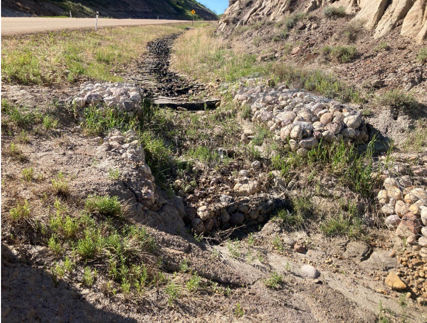
Photo 2 Gully erosion downstream of the gabion baskets (indicated by red arrow) is in similar condition since the 2021 inspection. Photo taken May 30, 2022, facing southeast.
