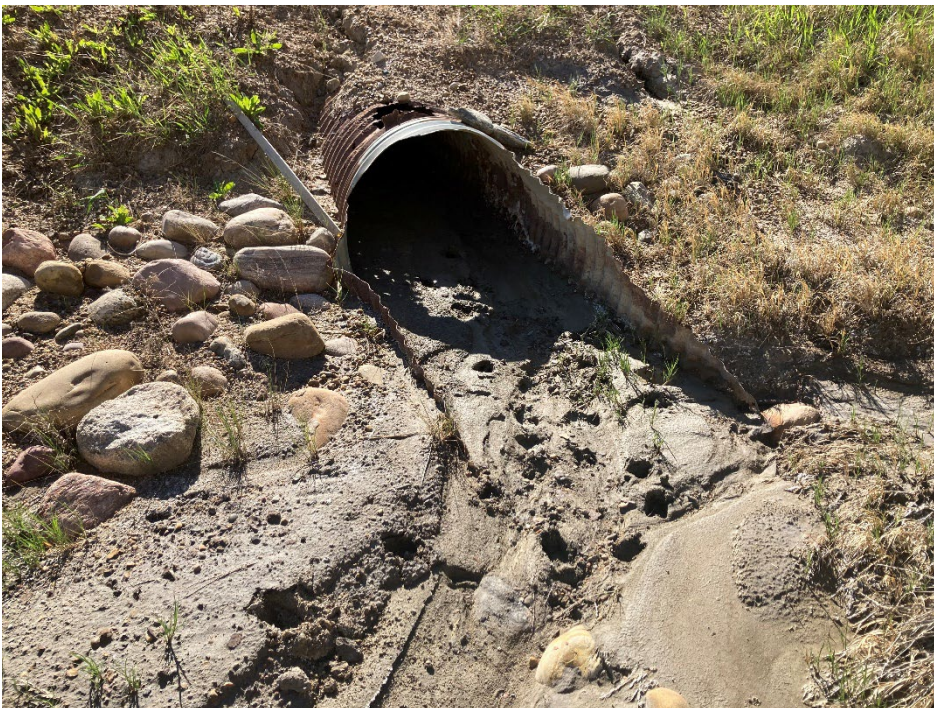
Photo 4 The CSP culvert underlying Hwy 837 (oriented east to west) is corroding and appears to be in similar condition as during the 2021 inspection. Photo taken May 30, 2022, facing northwest.
