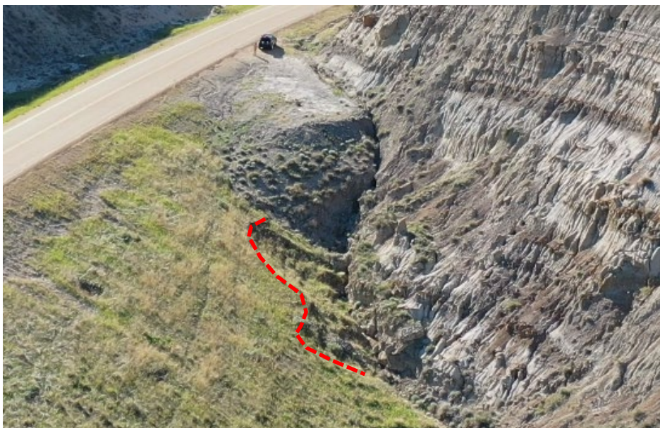
Photo 6 Slope failure triggered by gully erosion at the toe of the slope north of Hwy 837 doesn't appear to have changed since the 2021 inspection. Photo taken May 30, 2022, facing northwest.
