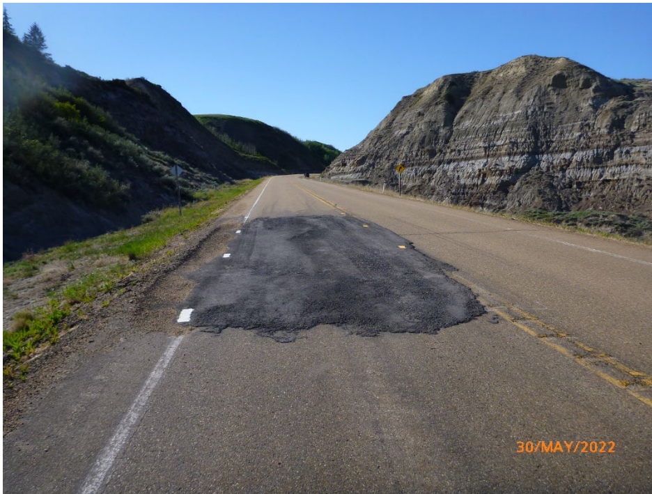
Photo 6 Slope failure triggered by gully erosion at the toe of the slope north of Hwy 837 doesn't appear to have changed since the 2021 inspection. Photo taken May 30, 2022, facing northwest.
