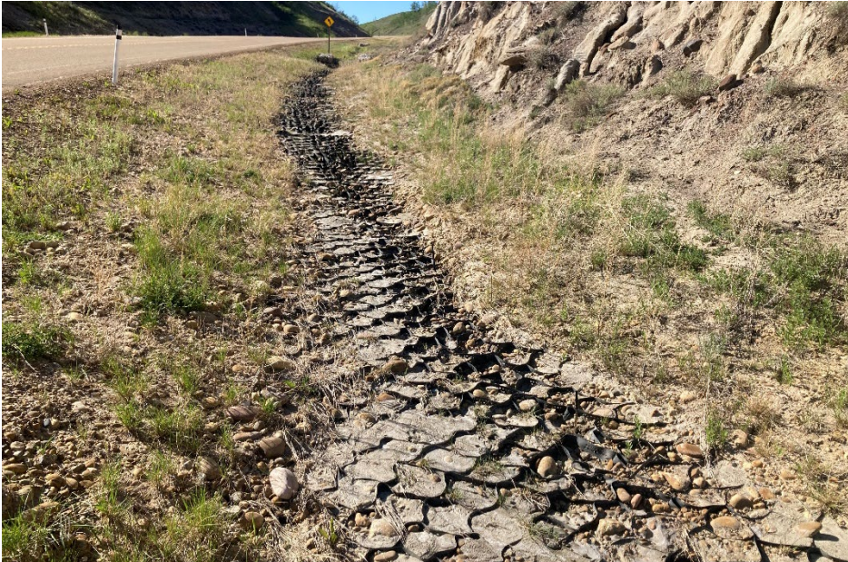
Photo 4 The CSP culvert underlying Hwy 837 (oriented east to west) is corroding and appears to be in similar condition as during the 2021 inspection. Photo taken May 30, 2022, facing northwest.
