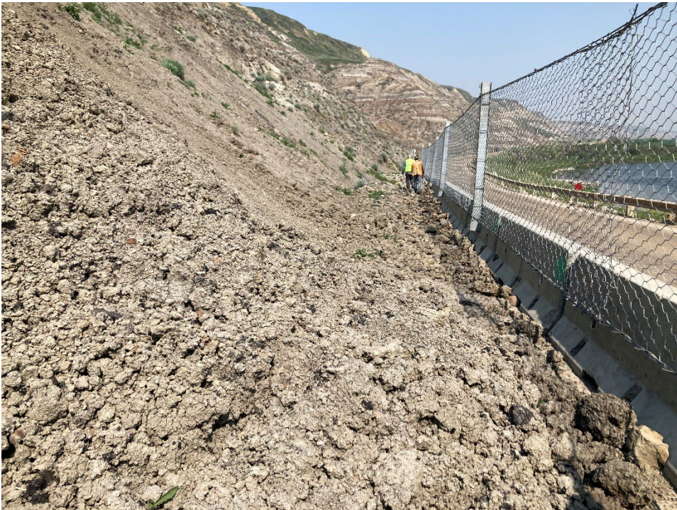
Photo 4 Material accumulating behind the jersey barrier and rockfall fence along C018-2. Photo taken June 10, 2025, facing northwest.
