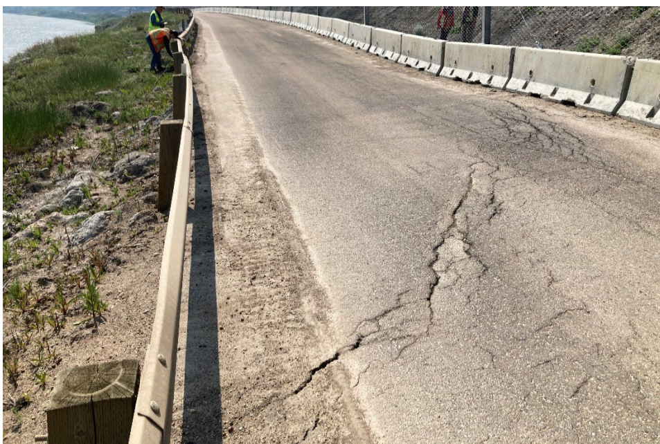
Photo 8 Pavement distress (settlement and cracking) near the northwest extent of the C018-2 site. The settlement has worsened between the 2024 and 2025 inspections and there is a significant dip in the east (northbound) lane. Photo taken June 10, 2025, facing south.
