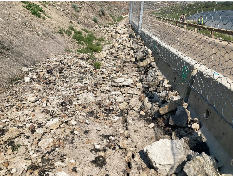
Photo 6 Pavement crack near the northwest extent of C018-2 appears wider (up to approximately 75 mm wide) than during the 2024 inspection when it was first observed. Photo taken June 10, 2025, facing northwest.
