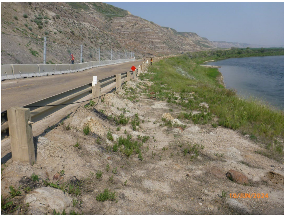
Photo 10 Material that has accumulated along the crest of the riverbank on the east side of the highway. Photo taken June 10, 2025, facing northwest.
