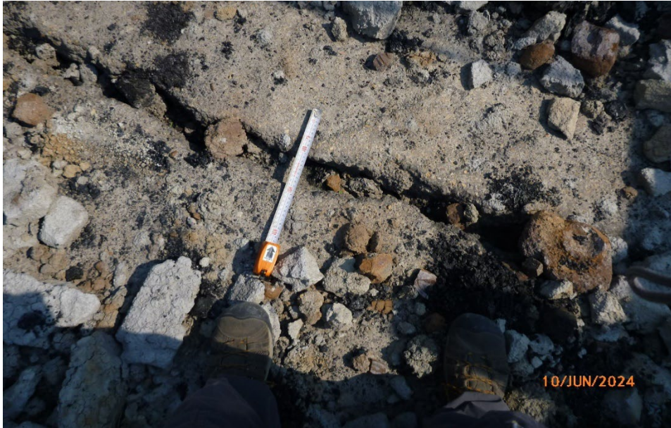
Photo 8 Pavement distress (settlement and cracking) near the northwest extent of the C018-2 site. The settlement has worsened between the 2024 and 2025 inspections and there is a significant dip in the east (northbound) lane. Photo taken June 10, 2025, facing south.
