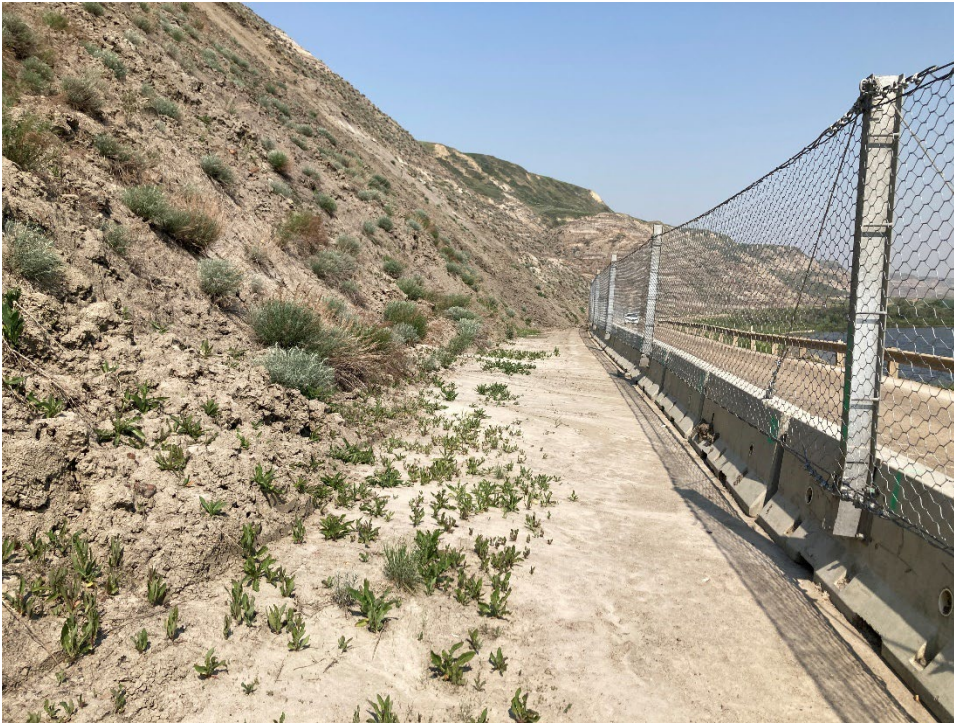
Photo 4 Material accumulating behind the jersey barrier and rockfall fence along C018-2. Photo taken June 10, 2025, facing northwest.
