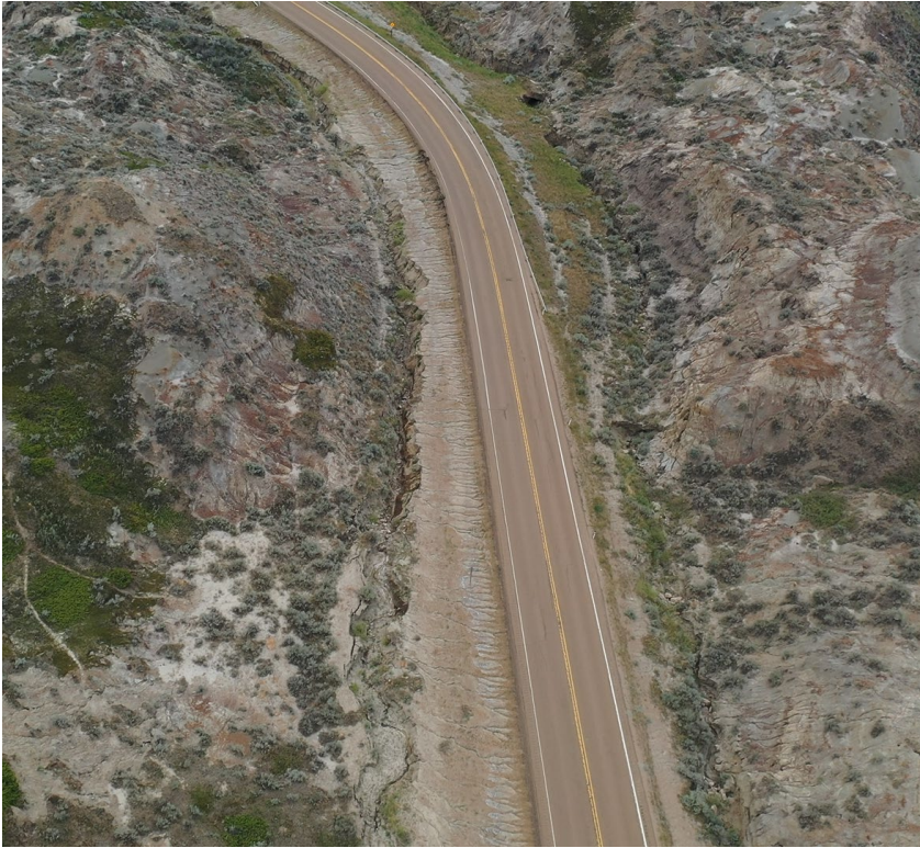
Figure 4 Oblique air photo of the highway highlighting the erosion gullies and rilling erosion along the north and south embankments. Photo taken August 16, 2021, facing east.
