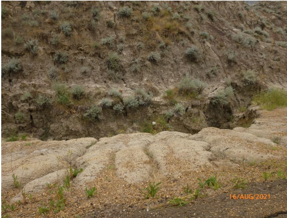
Figure 6 Large gullies and rilling erosion along the embankment slope. Photo was taken August 16, 2021, facing south.
