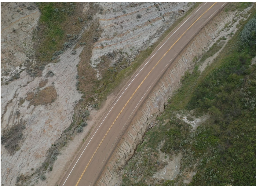
Figure 4 Oblique air photo of the highway highlighting the erosion gullies and rilling erosion along the north and south embankments. Photo taken August 16, 2021, facing east.
