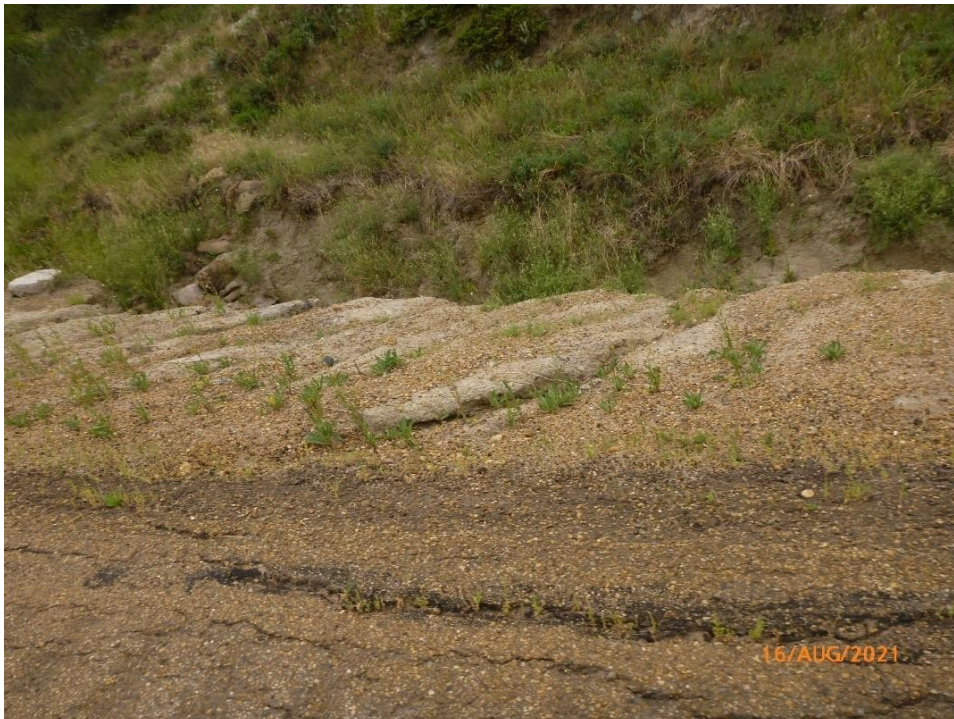
Figure 6 Large gullies and rilling erosion along the embankment slope. Photo was taken August 16, 2021, facing south.
