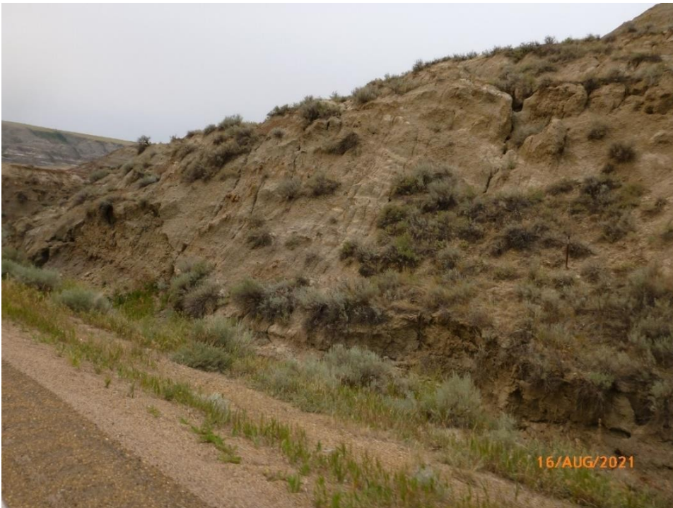
Figure 8 North natural slope eroding into the ditch. Photo was taken on August 16, 2021, facing north-west.
