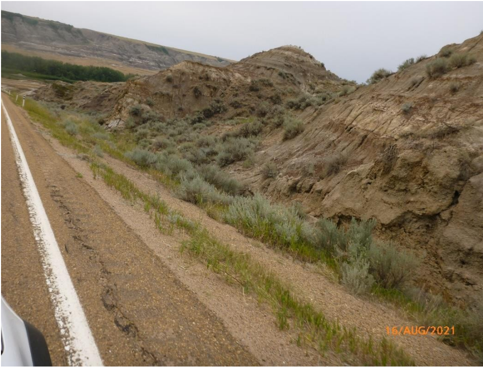
Figure 8 North natural slope eroding into the ditch. Photo was taken on August 16, 2021, facing north-west.
