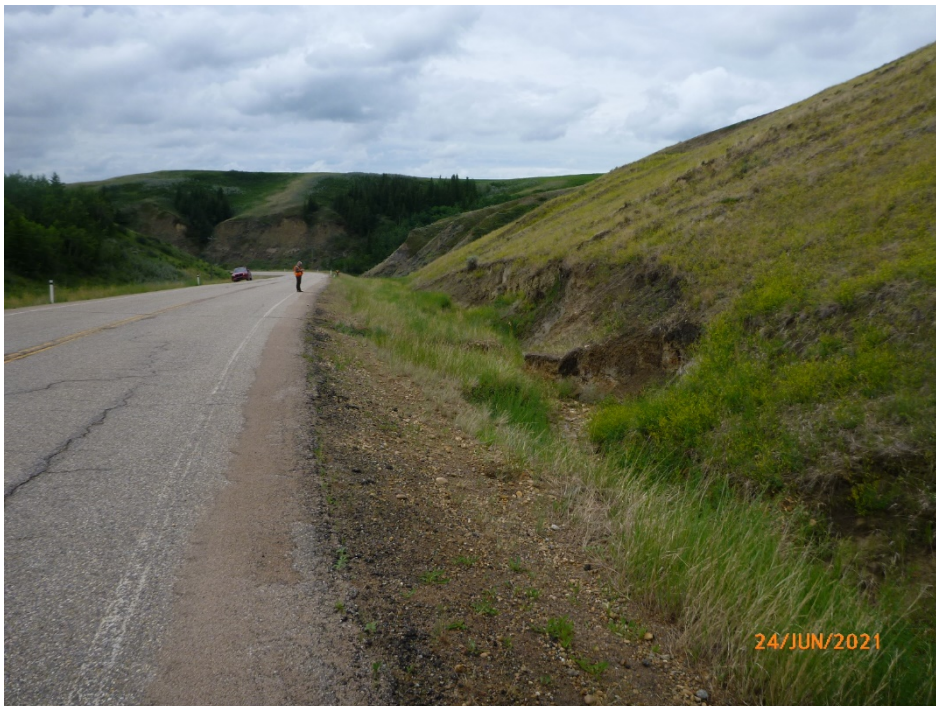
Photo 6 Ongoing erosion of the toe of the slope west of Hwy 841. Photo taken June 24, 2021 facing southwest.
