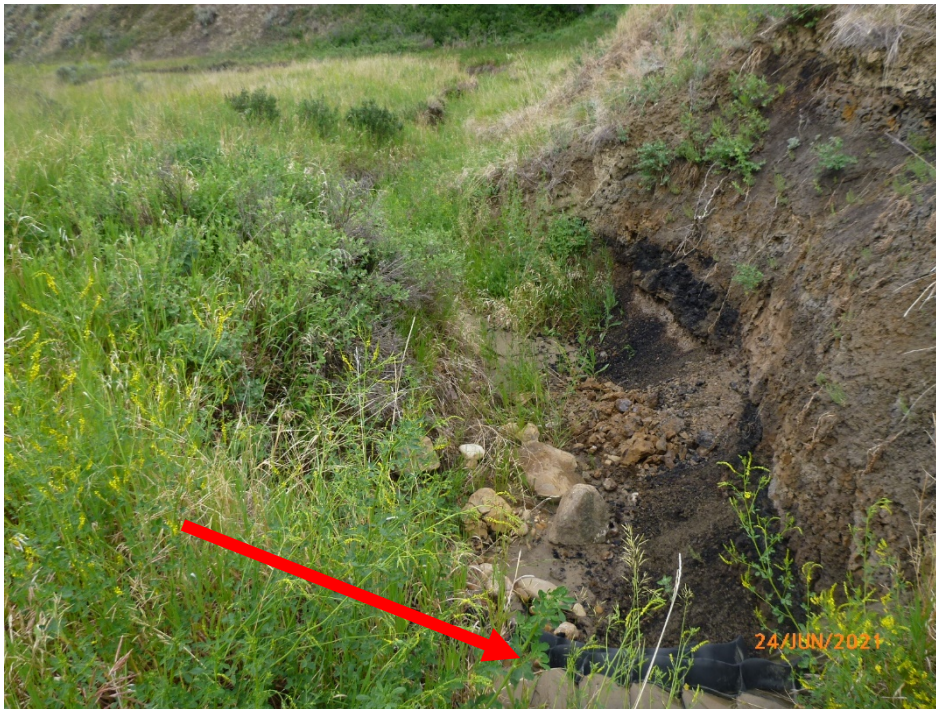
Photo 6 Ongoing erosion of the toe of the slope west of Hwy 841. Photo taken June 24, 2021 facing southwest.
