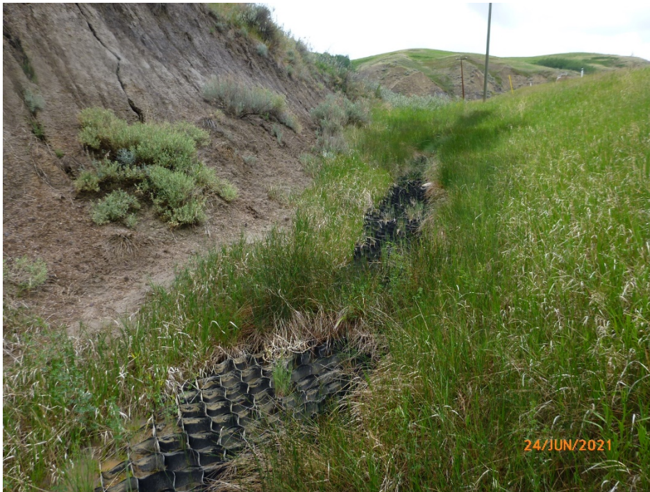
Photo 4 An embankment slope failure observed on the west (southbound) portion of the highway embankment slope, upslope of the gully erosion and near the south extent of the site. Photo taken June 24, 2021 facing southwest.
