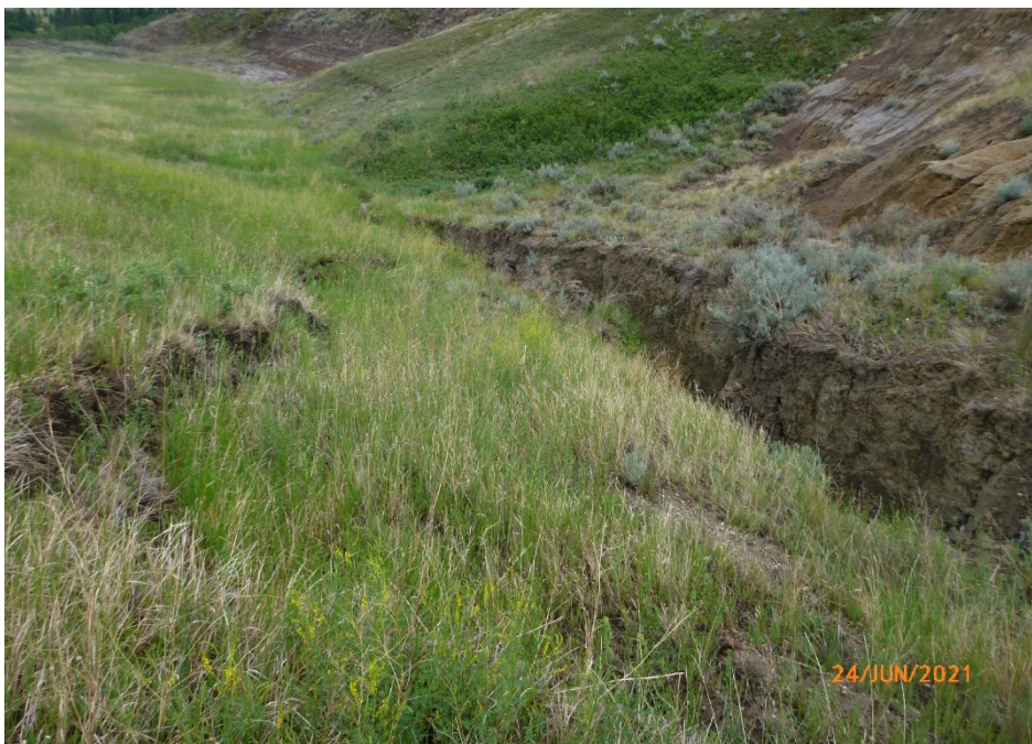
Photo 4 An embankment slope failure observed on the west (southbound) portion of the highway embankment slope, upslope of the gully erosion and near the south extent of the site. Photo taken June 24, 2021 facing southwest.
