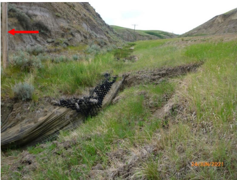
Photo 2 A failed section of geocell armouring that was previously installed near the south extent of the site. Red arrow indicates power pole that will be impacted by erosion. Photo taken June 24, 2021 facing north.
