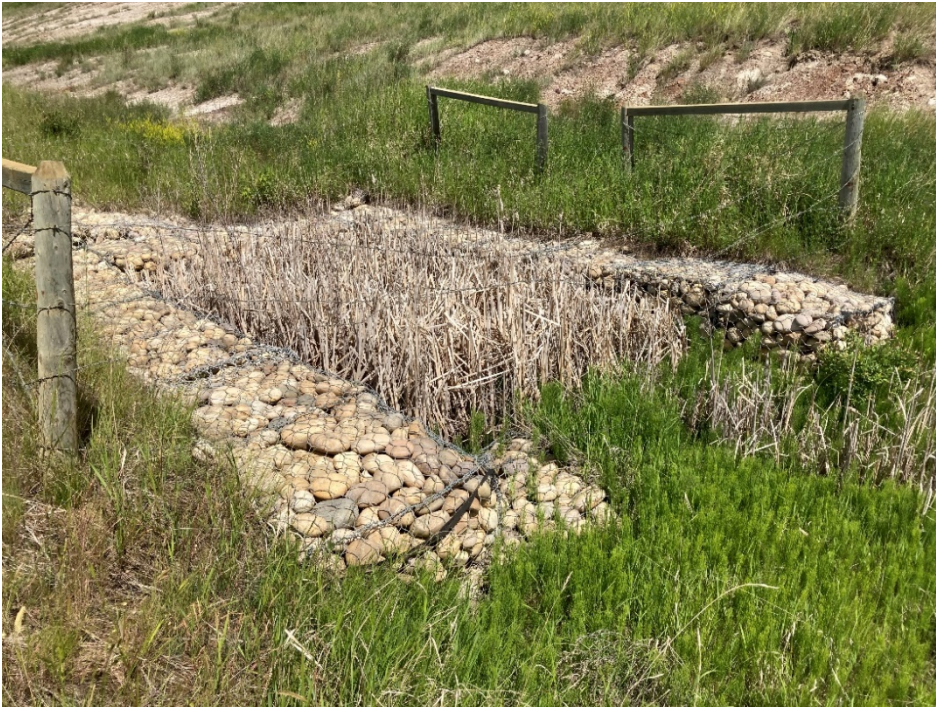
Photo 4 Sediment deposit from a previous high-water event at the outlet of the gabion mattress lined channel. Photo taken June 24, 2020 facing south.
