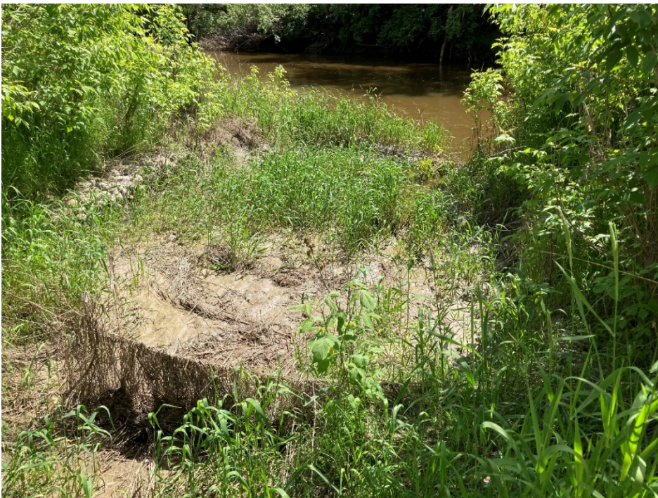
Photo 4 Sediment deposit from a previous high-water event at the outlet of the gabion mattress lined channel. Photo taken June 24, 2020 facing south.
