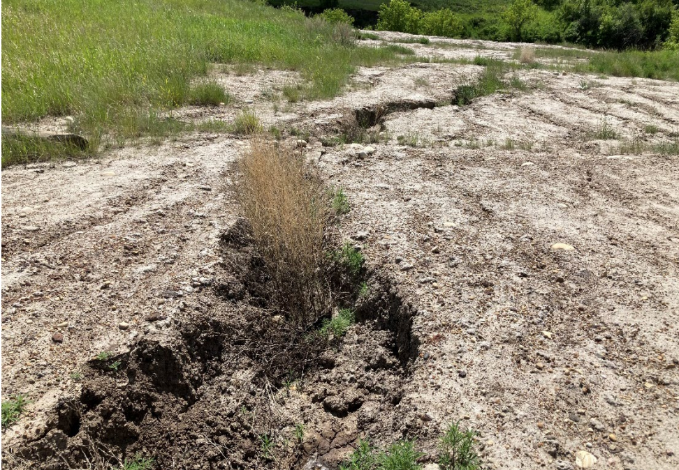
Photo 2 Vegetation and sediment build-up at the catch basin structure at the inlet of the culvert. Photo taken June 24, 2020 facing east.
