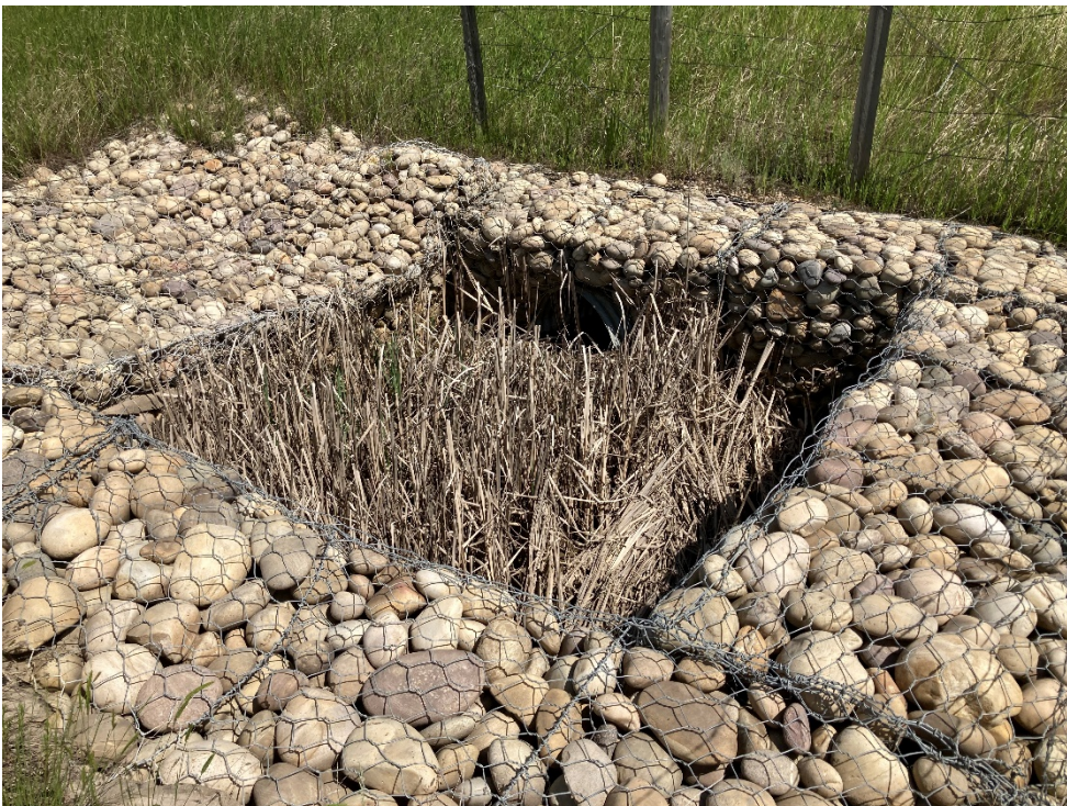
Photo 2 Vegetation and sediment build-up at the catch basin structure at the inlet of the culvert. Photo taken June 24, 2020 facing east.
