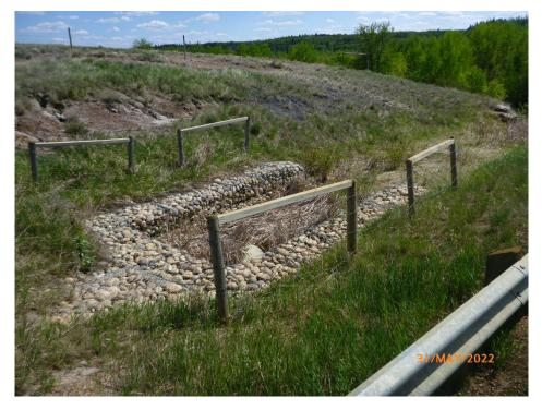
Photo 4 Failed section of the gabion mattress lined channel east of the highway. Photo taken May 31, 2022, facing northwest.
