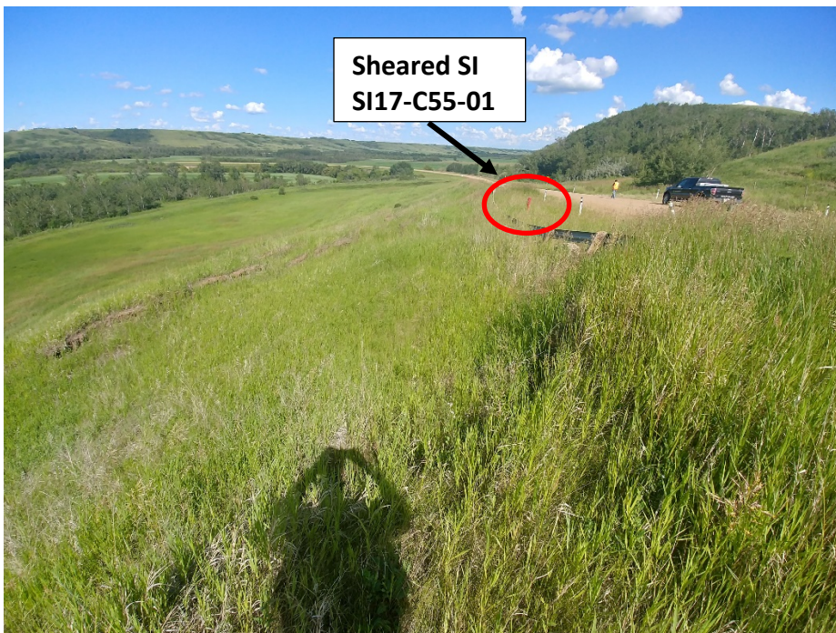
Photo 2 View of C055-I slide area, settled guardrail, and sheared SI. Photo taken July 12, 2019 looking east.
