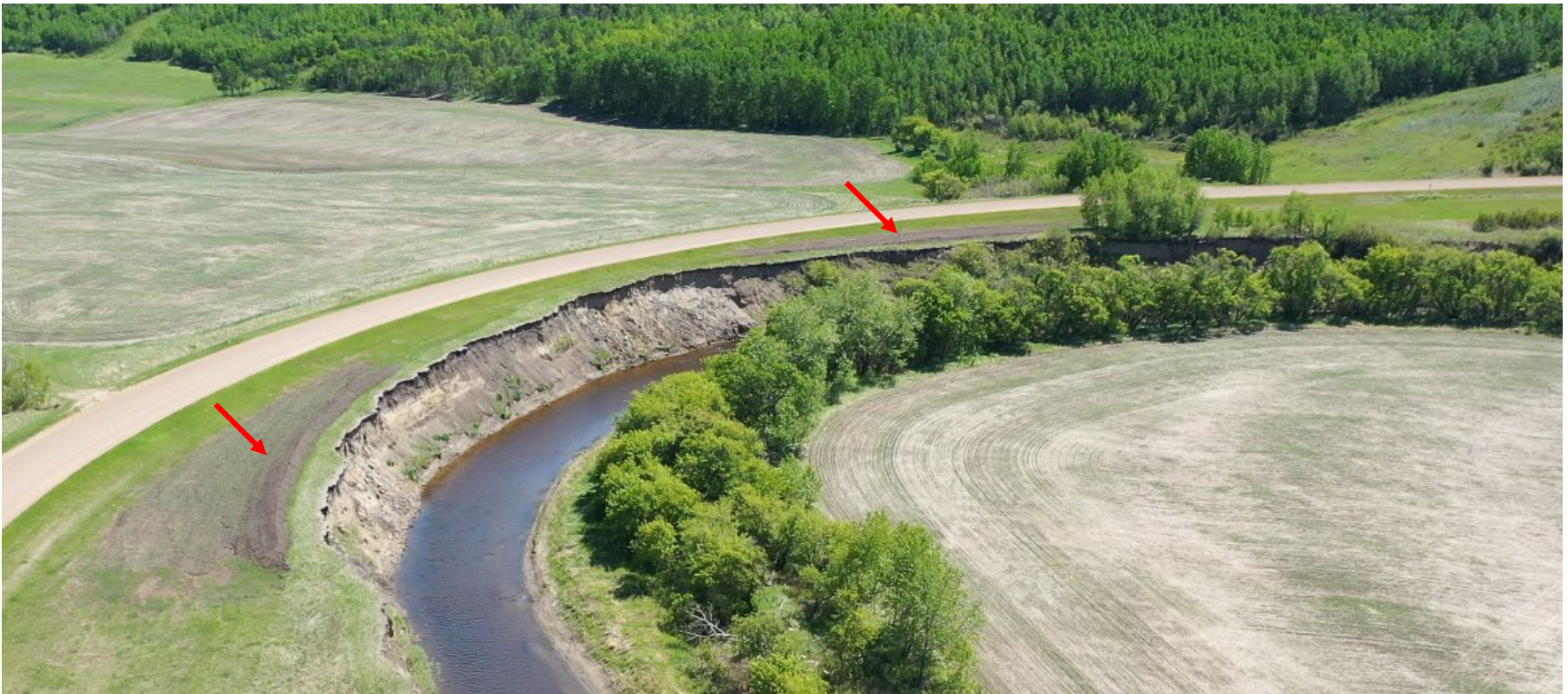
Photo 5 Aerial photo of the C055-II riverbank erosion. Two berms were constructed in late-2021 near the northeast and southwest extent of the riverbank erosion (indicated by the red arrows) in an attempt to divert flow in the west ditch away from the eroding bank. Photo taken May 31, 2022, facing south.
