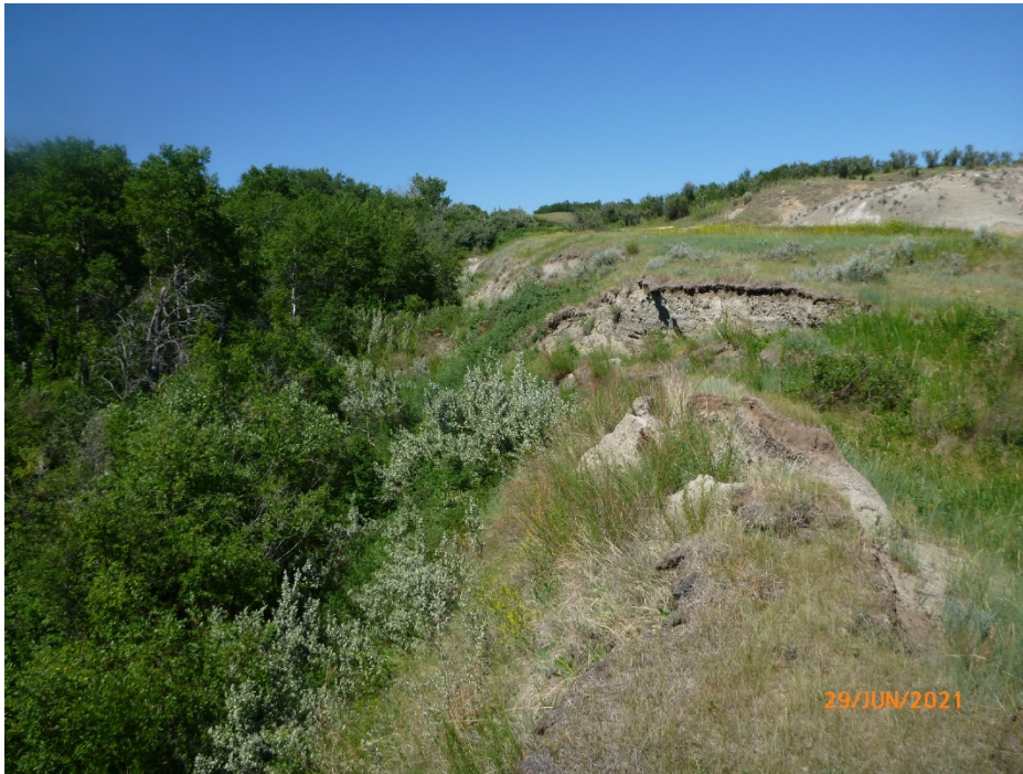
Photo 7 Ground cracking observed east of the eastern highway embankment (indicated by black arrow) and above the east gully slope. Photo taken June 29, 2021 facing southwest.
