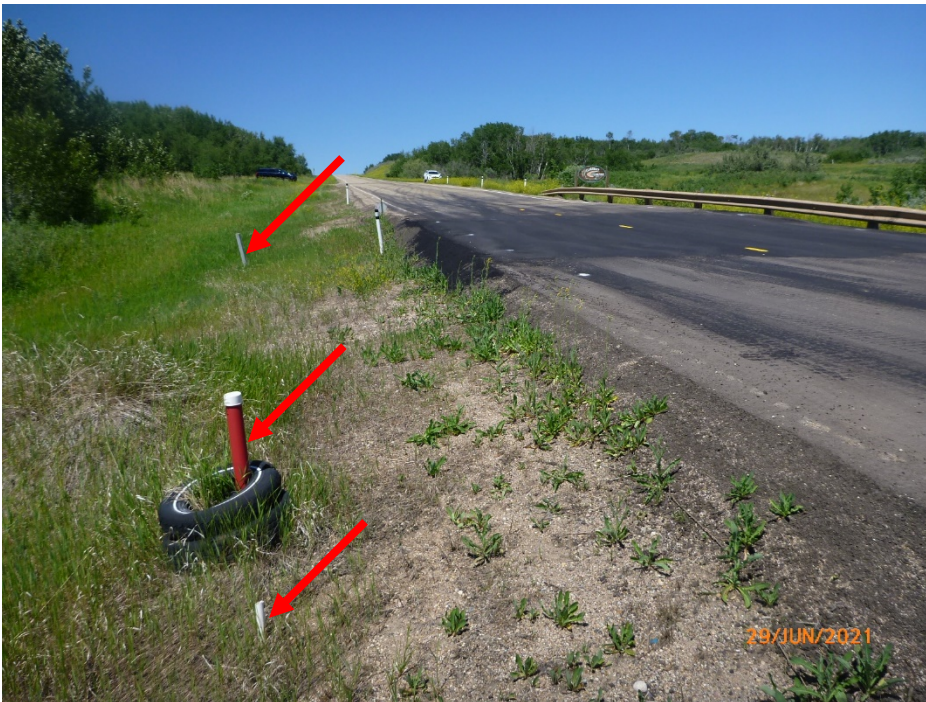
Photo 5 Guardrail deflection and a recent asphalt patch near the north extent of the site. The guardrail deflection is more severe in the west (southbound) guardrail. Photo taken June 29, 2021 looking south.
