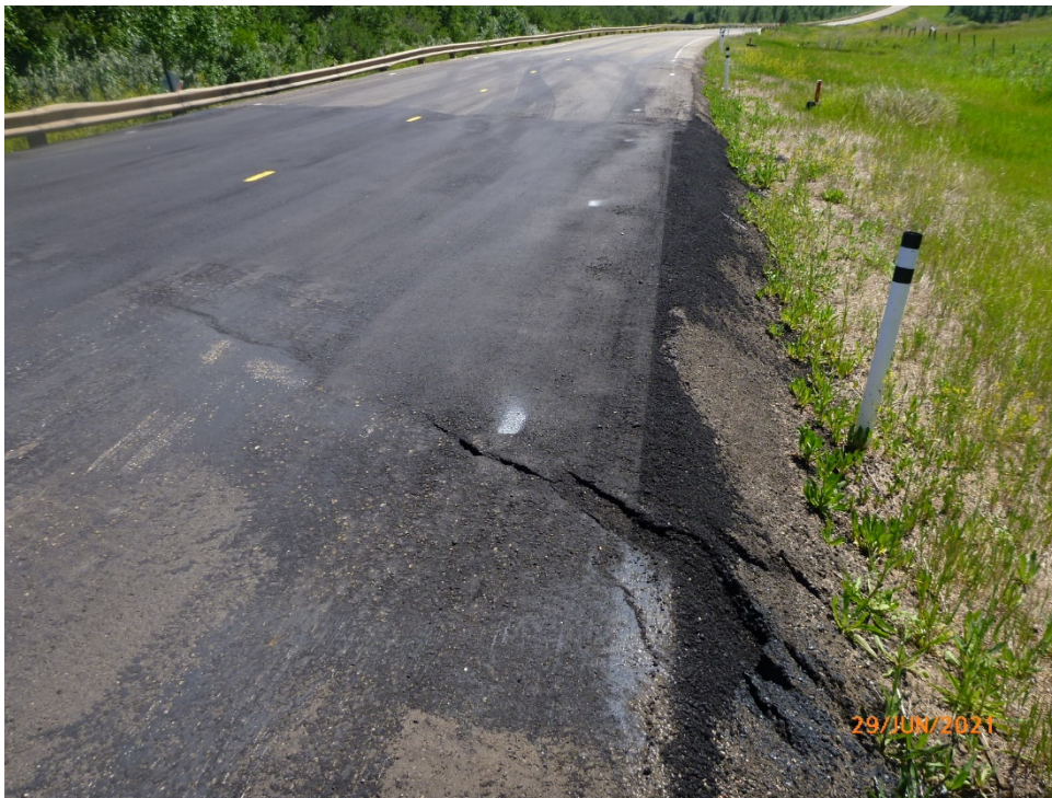
Photo 3 Transverse pavement cracking observed in a recent asphalt patch, on the north flank of slide. Photo taken July 12, 2019 looking south.
