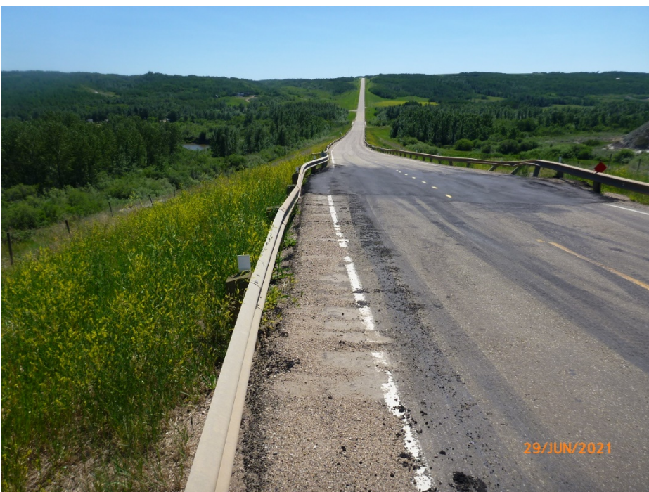
Photo 5 Guardrail deflection and a recent asphalt patch near the north extent of the site. The guardrail deflection is more severe in the west (southbound) guardrail. Photo taken June 29, 2021 looking south.
