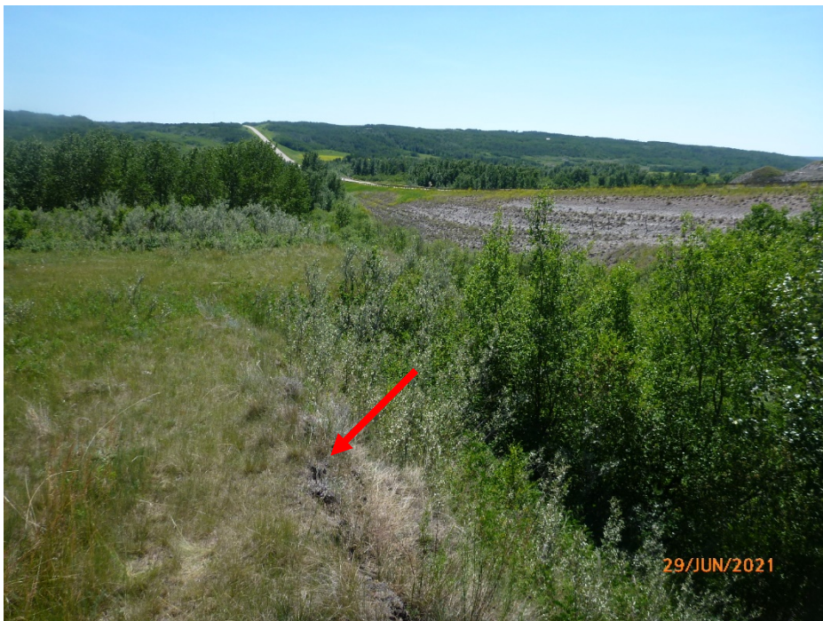
Photo 7 Ground cracking observed east of the eastern highway embankment (indicated by black arrow) and above the east gully slope. Photo taken June 29, 2021 facing southwest.
