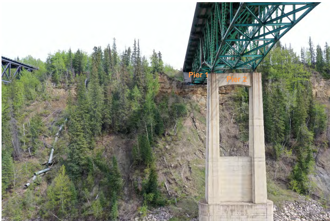
Photo 2: Gullies downslope of east abutment and broken culvert north of east embankment. Facing southeast.
