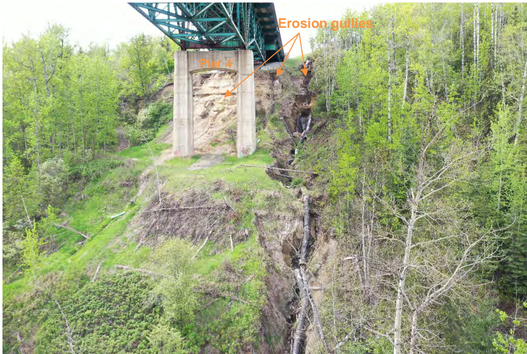
Photo 6: Broken culvert and gully on the north side of the west abutment. Looking northwest.
