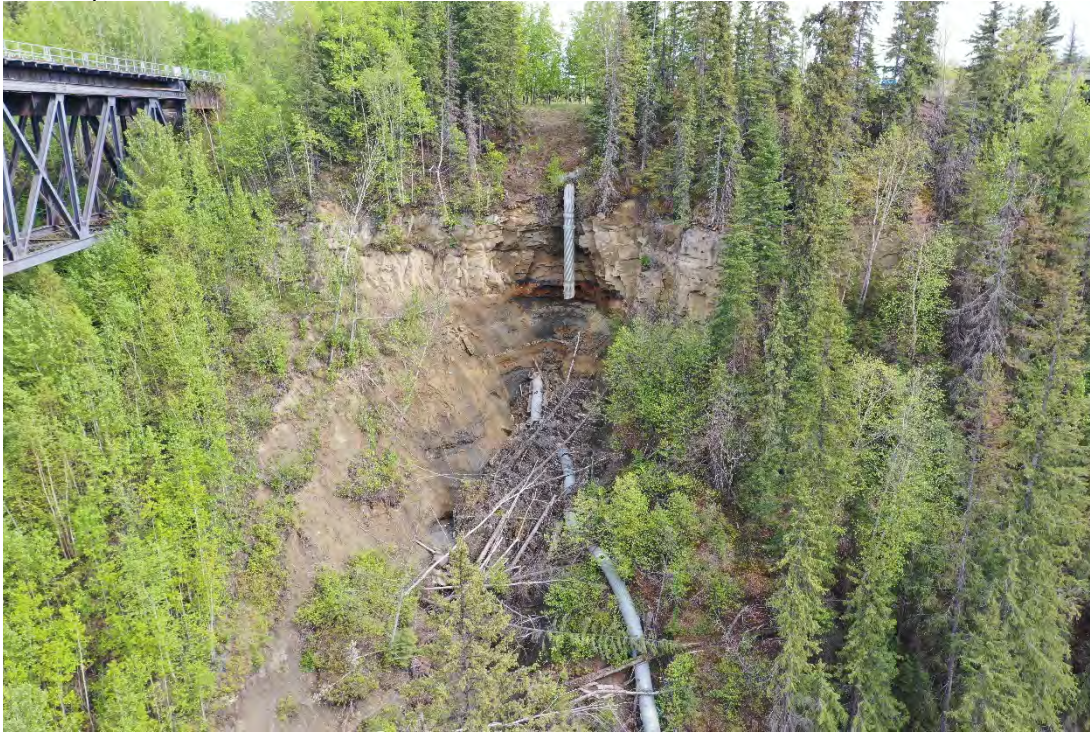
Photo 9: Broken culvert north from the east bridge abutment. Facing southeast.
