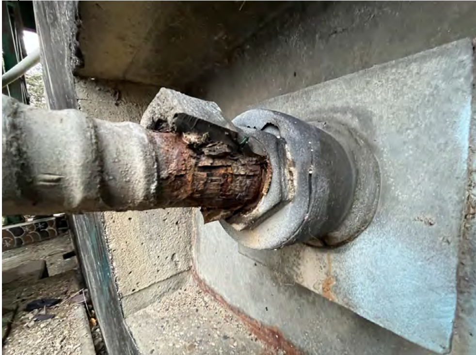
Photo 11: Corroded soil anchor on east abutment. Photo taken by Stantec bridge team, November 14, 2024.
