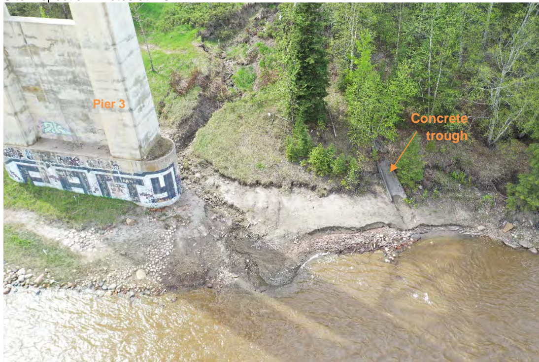
Photo 7: Erosion gully next to west pier at river level, facing west.
