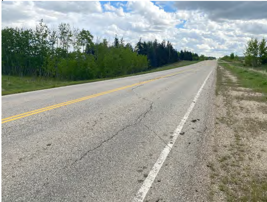
Photo 3: North limits of semi-circular crack. Looking southeast.
