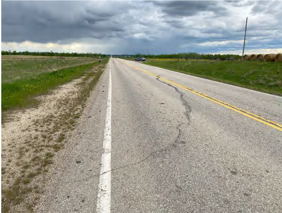
Photo 1: South limits of semi-circular crack. Looking north.
