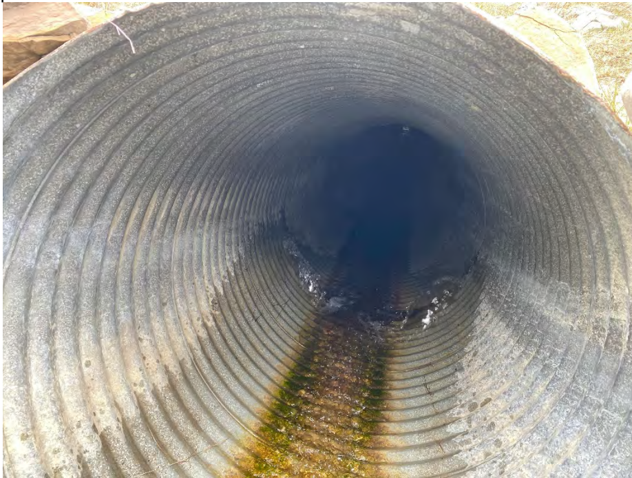
Photo 13: Water undermining west culvert inlet and entering between the first and second culvert segments at the culvert site. Looking northeast.
