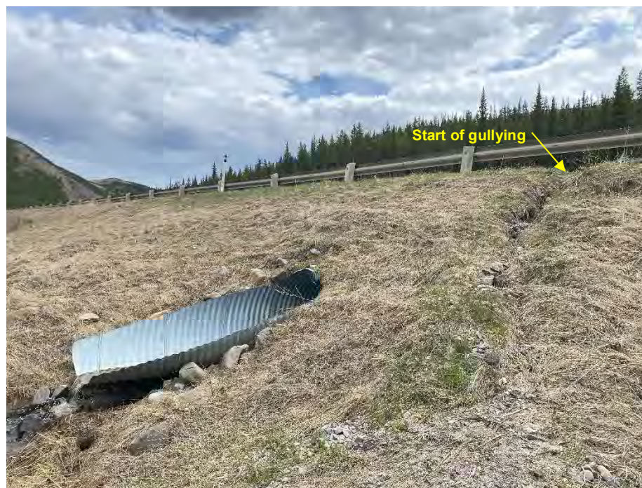
Photo 2: Gully on north side of the highway and undermining of C/L culvert outlet. Looking southeast.
