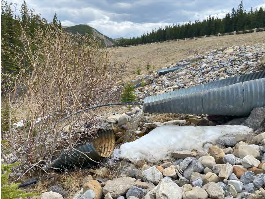
Photo 9: Water undermining culvert, which has slid further downslope. Looking east.
