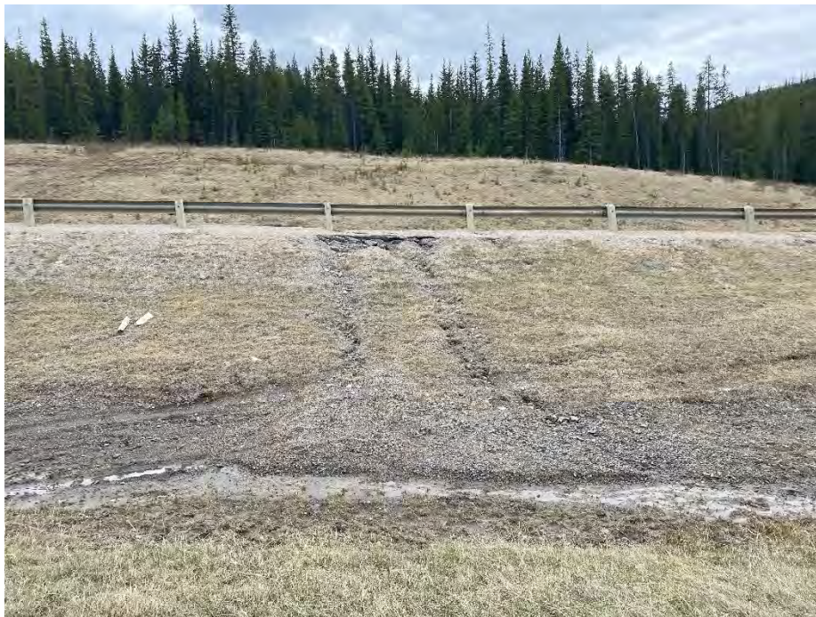
Photo 6: Seepage along north ditch between pile wall site and culvert site with erosion rills and gully on the north ditch highway shoulder. Looking south.
