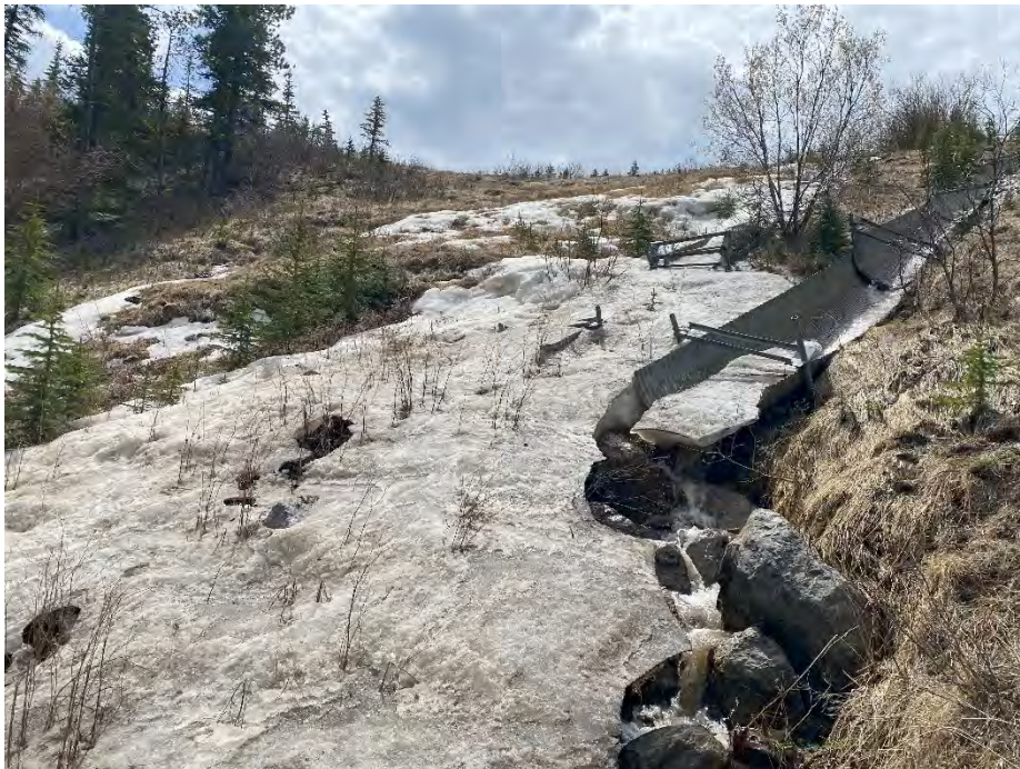
Photo 10: Twisted bracing along half-round culverts, east culvert under snow. Looking south.
