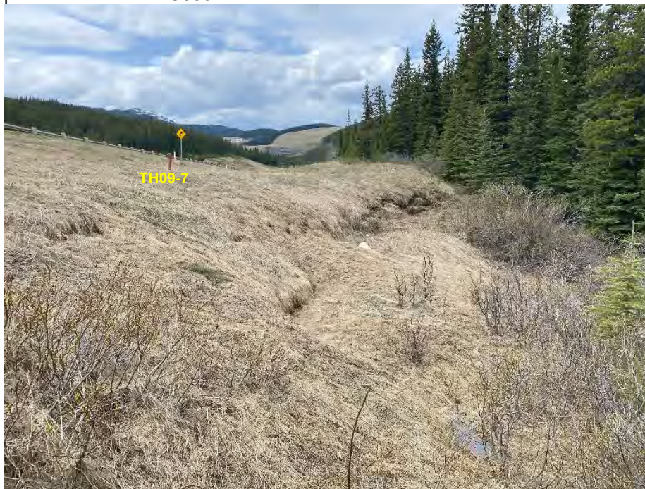
Photo 1: Retrogressive scarp on the north side of the pile wall, looking west.
