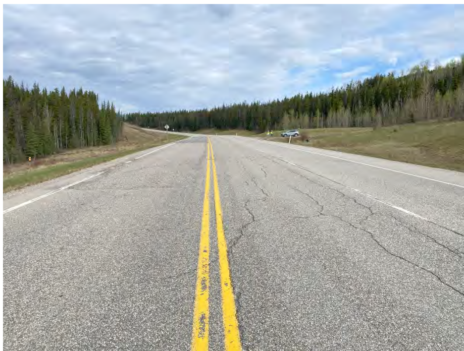
Photo 4: Curved cracks extending further south. Looking northwest.
