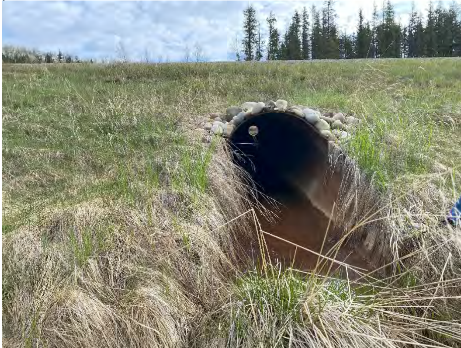
Photo 7: Vegetation blocking C/L culvert outlet. Looking northeast.
