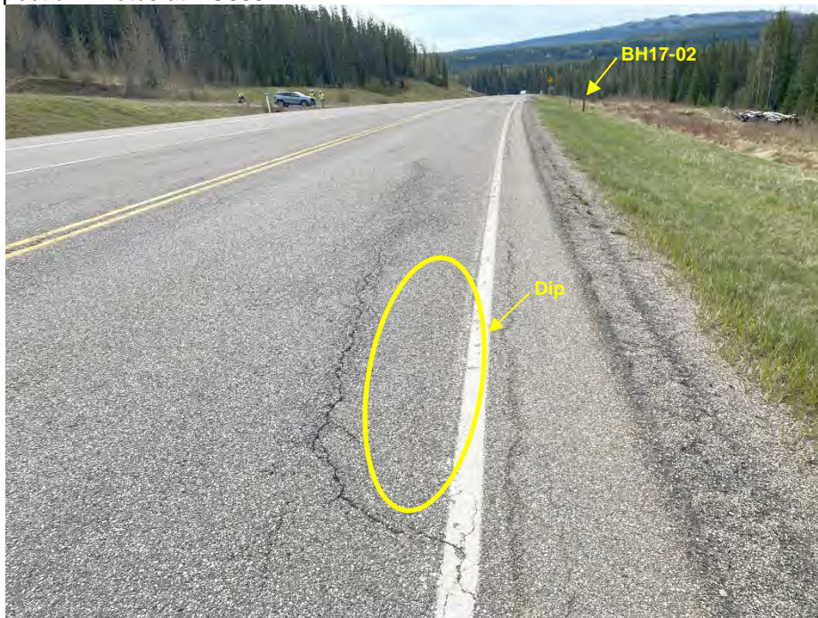
Photo 3: New cracking and ~10 mm dip in SBL northwest from BH17-02 and north from vehicle tracks with seepage. Looking southwest.
