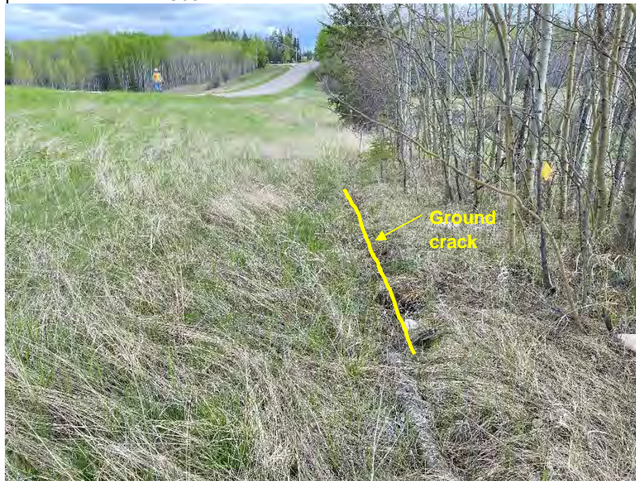
Photo 5: South ditch, looking east. Ground crack visible near fence line, possibly due to removal of silt fence.
