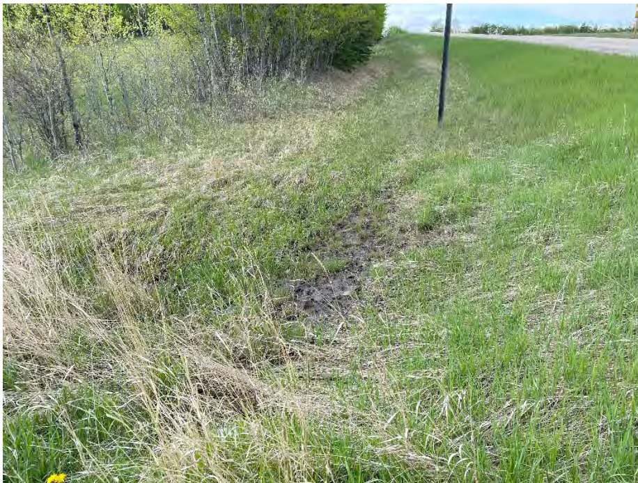
Photo 4: Erosion at west end of culvert across property access road. Looking west.
