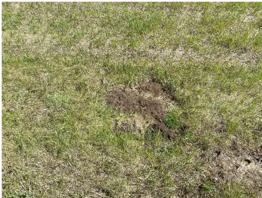
Photo 8: Sinkhole backfilled with soil, southeast from the utility box in the east ditch near the mid-hill landslide area. Looking north.
