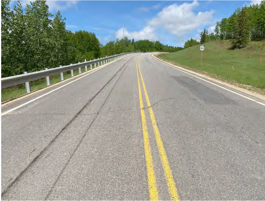
Photo 3: Cracks reflecting through pavement repair at south extent of mid-slope landslide. Looking northwest.
