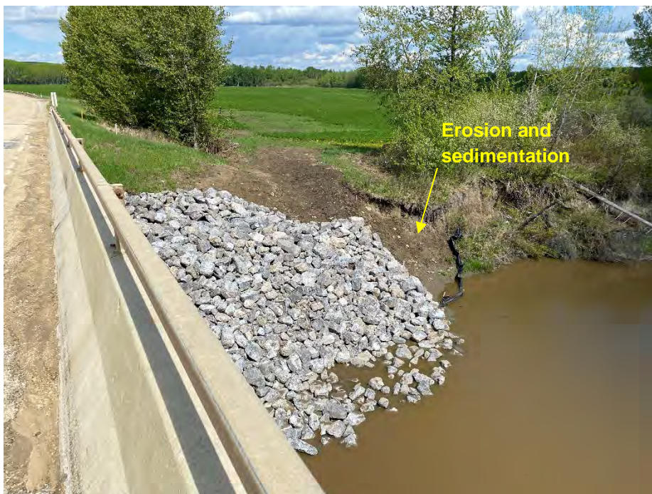
Photo 8: East side repair with riprap at north abutment. Looking northeast.
