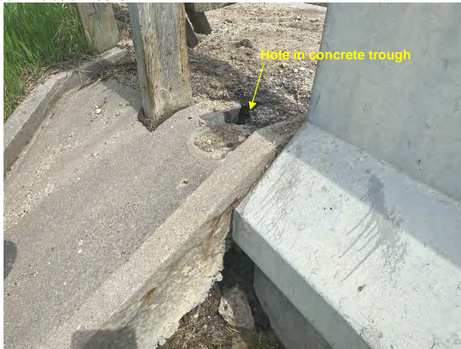
Photo 5: Hole in concrete trough at northwest bridge abutment allowing water to drain through. Facing northeast.
