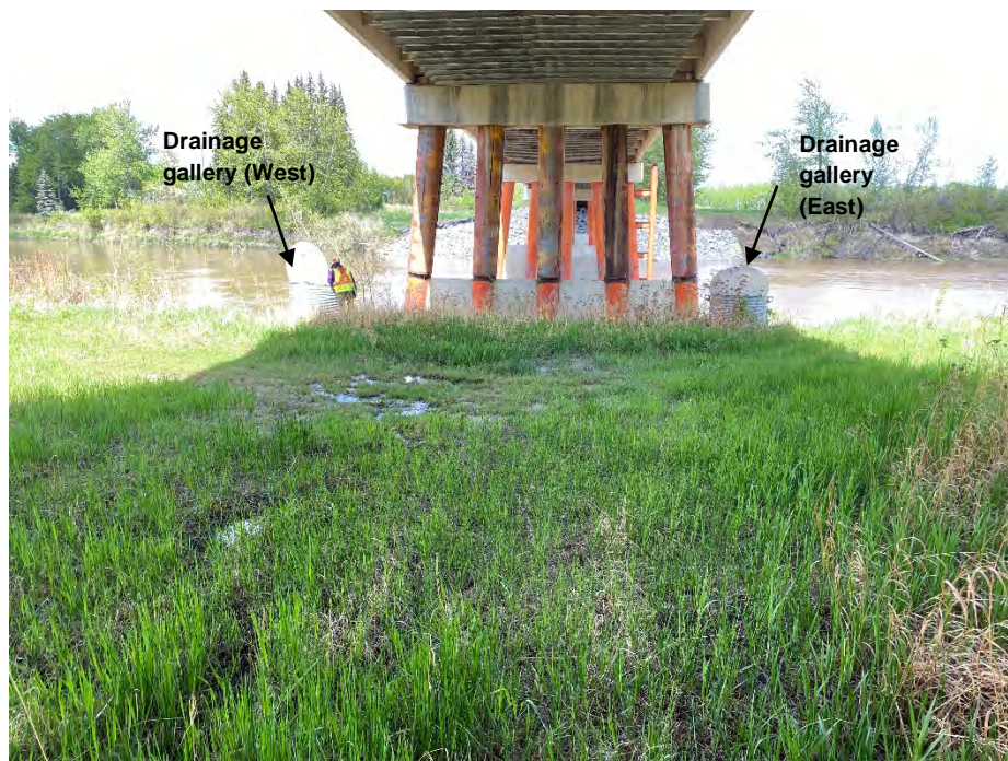
Photo 14: Saturated ground between drainage galleries and Pier 1. Looking northeast.
