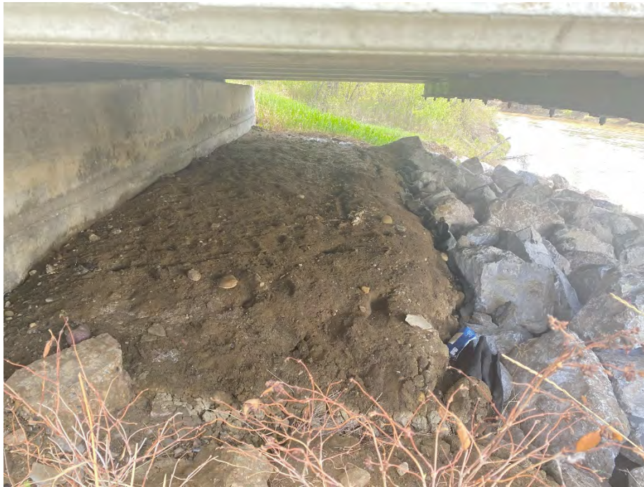
Photo 7: North abutment head slope repaired and armoured with riprap. Looking southeast.
