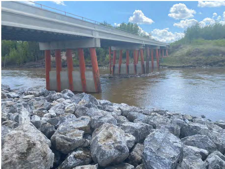
Photo 6: Few driftwood present, north headslope armoured with riprap. Looking south.
