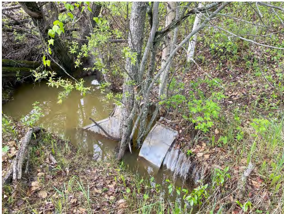
Photo 6: Separation at 900 mm diameter culvert inlet. Looking southwest.
