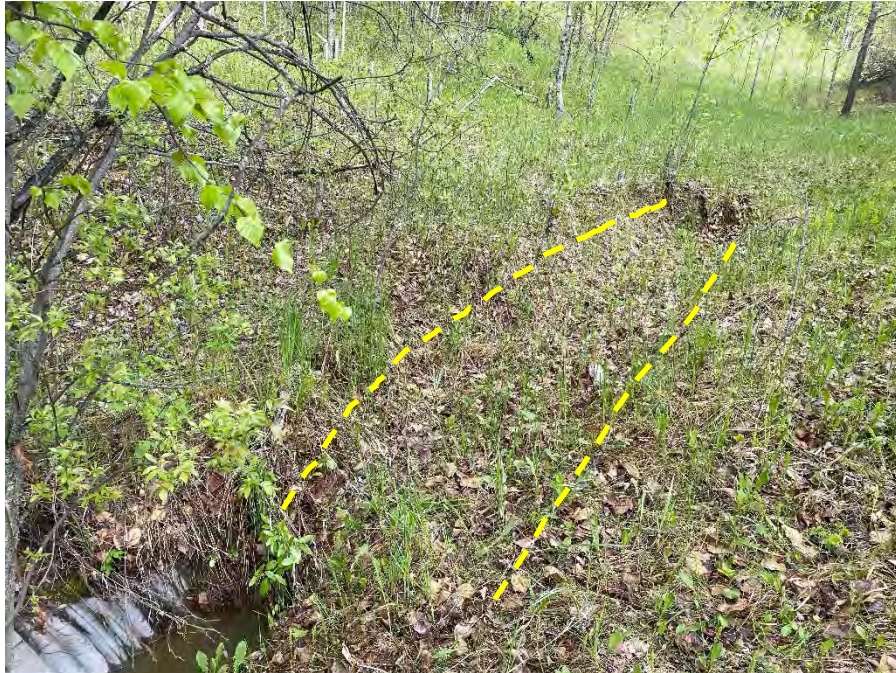
Photo 7: Subsidence along culvert alignment. Looking northwest.
