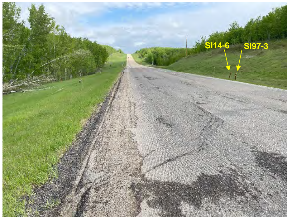
Photo 2: South end of landslide pavement cracking. Looking north.
