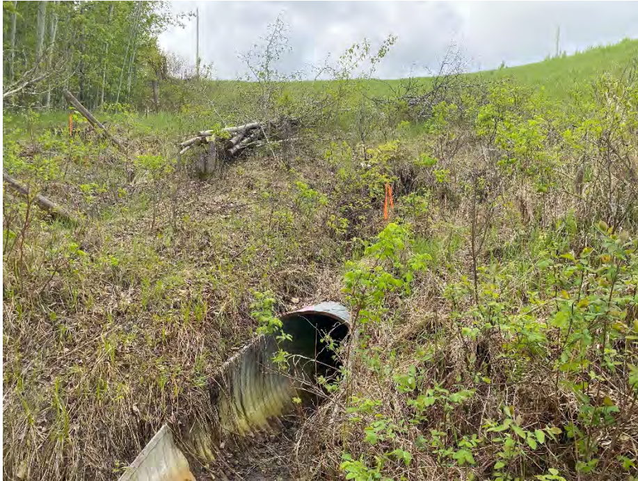
Photo 9: Culvert outlet and settlement above culvert. Looking southeast.
