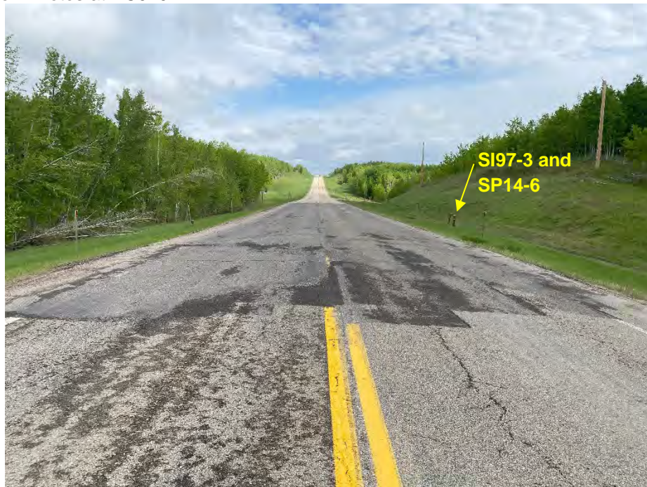
Photo 1: South end of milled / patched highway area. Looking north.
