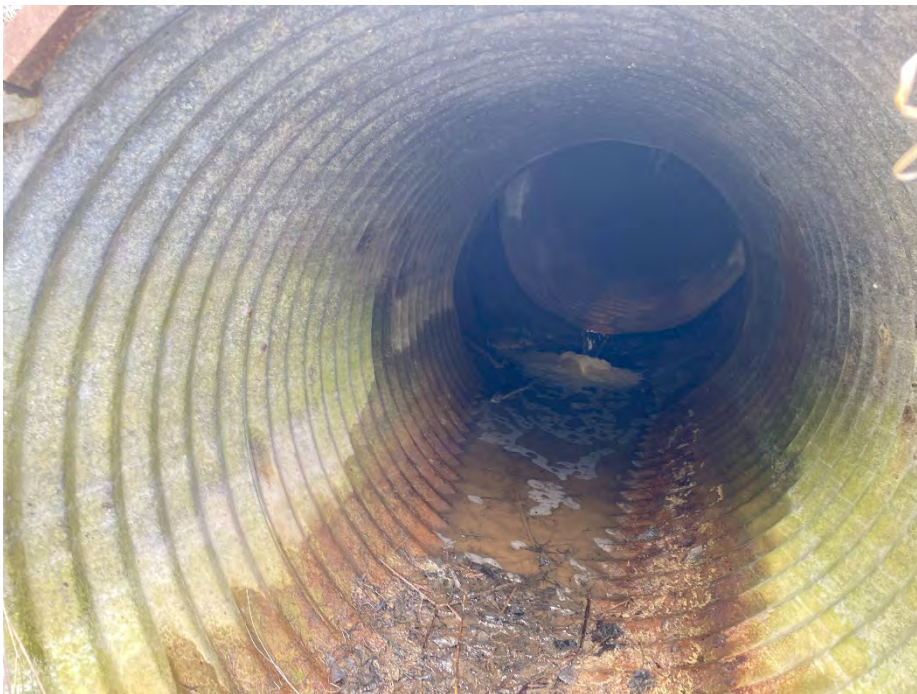
Photo 10: Separation at first joint from culvert outlet. Looking southeast.
