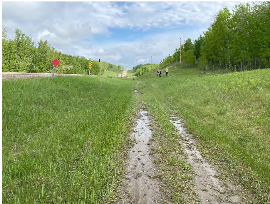
Photo 4: Flowing water and sedimentation in wheel tracks on east side of highway, south from backslope slump #3. Looking north.
