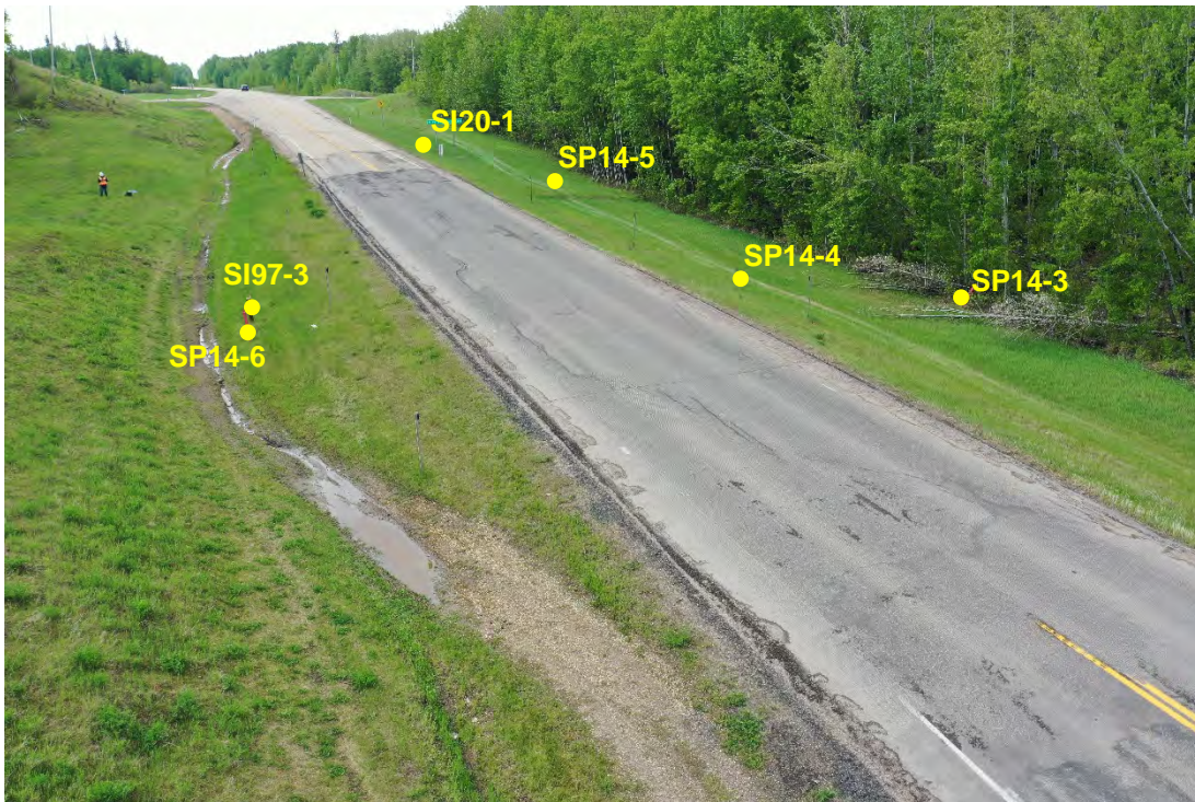
Photo 12: Aerial view of pavement cracking, taken by drone. Facing southwest.
