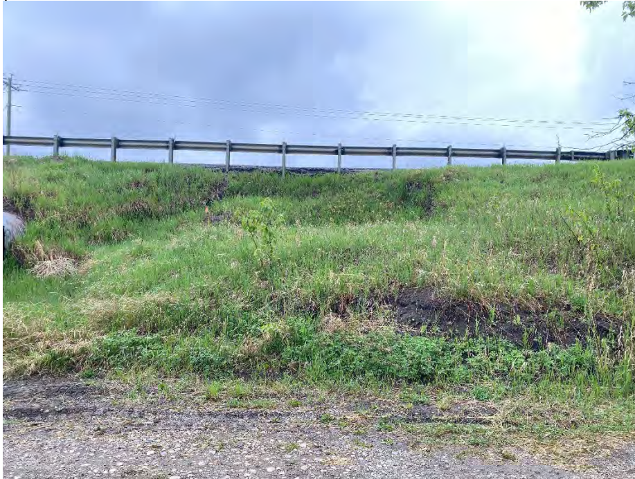
Photo 1: Slump on east side of culvert. Looking north.
