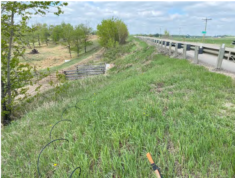
Photo 2: Slump across cattlepass culvert. Looking west.
