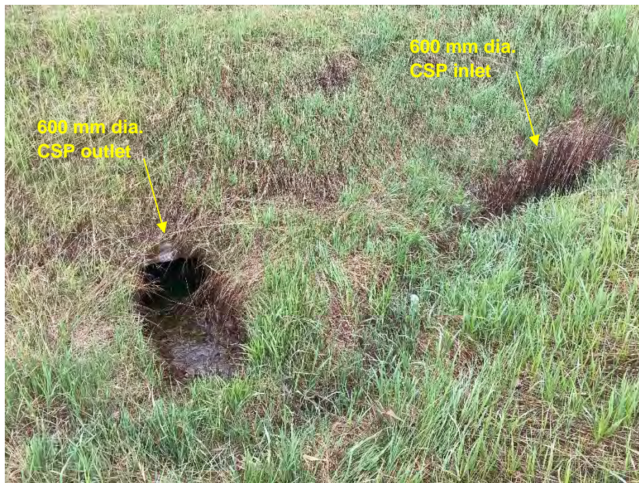
Photo 10: Water ponded in sunken culvert outlet in ditch east of private access, north side of highway. Looking south.
