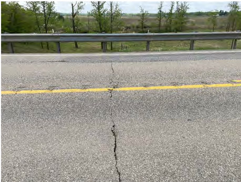
Photo 6: Transverse pavement crack above cattlepass culvert. Looking south.
