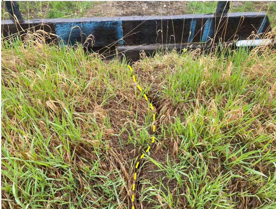
Photo 7: Ground crack along centreline of cattlepass culvert at north end. Looking north.
