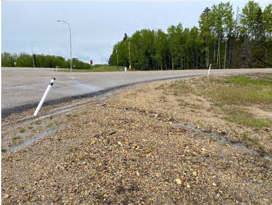
Photo 7: Erosion occurring off the east corner of Hwy 759 and Hwy 39, into the north ditch. Looking west.
