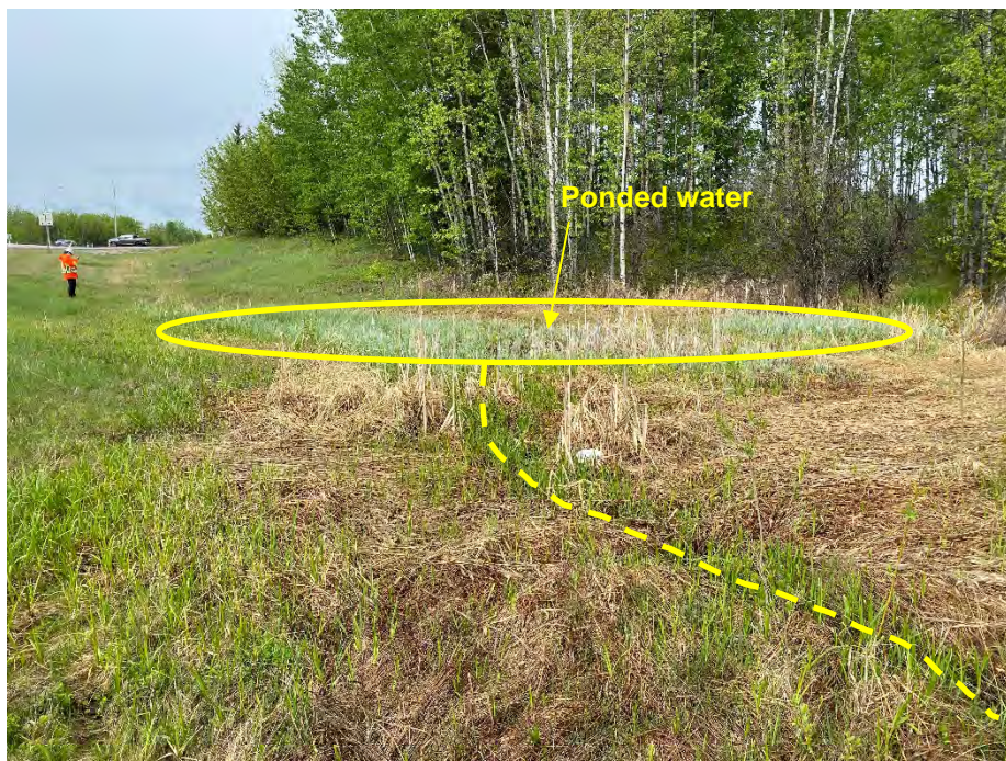
Photo 8: Ponded water located in the north ditch, water flowing towards east. Facing southwest.
