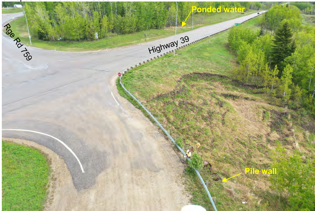
Photo 9: Aerial view of the slide and surrounding pavement. Taken by drone, facing northeast.
