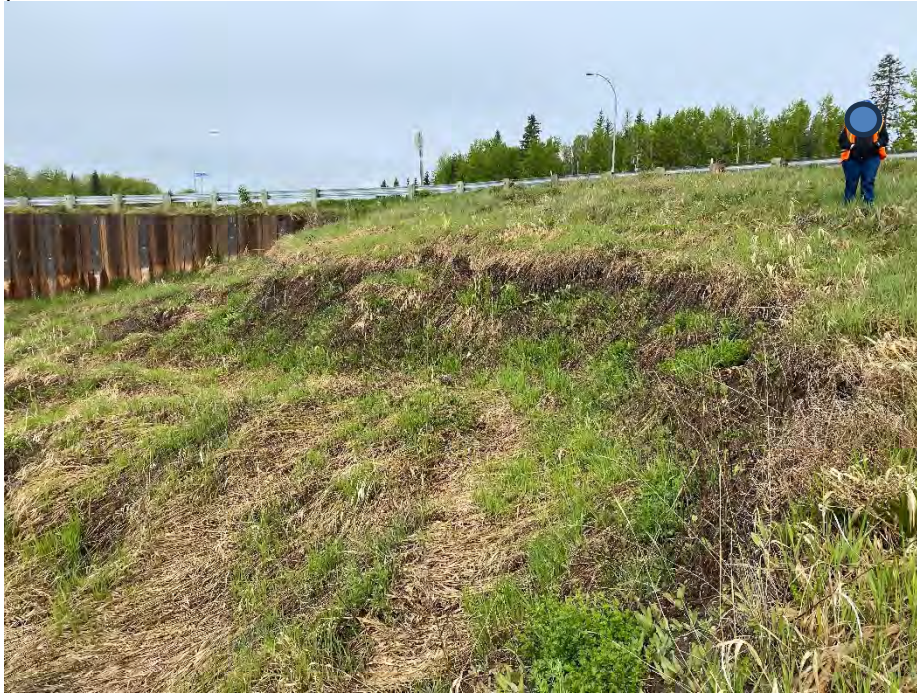
Photo 3: Scarp less vegetated than previous inspection. Looking northwest.
